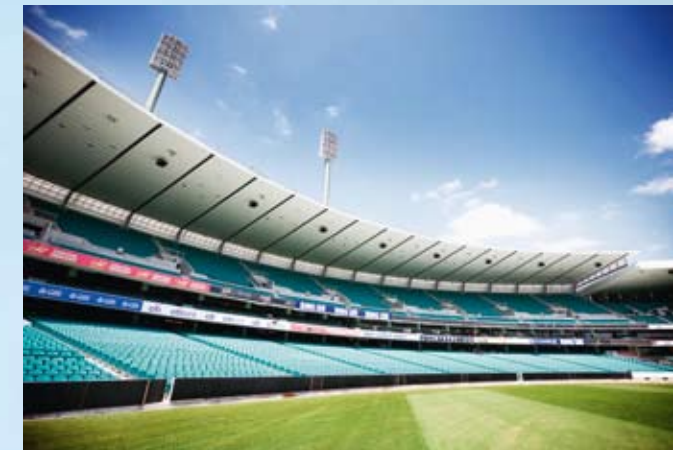
STATE-OF-THE-ART: Work has been completed on the new $70 million Victor Trumper Stand at the SCG. It will be unveiled to AFL football in round four, 2009, when the Sydney Swans play Carlton in a historic first Saturday afternoon clash.
