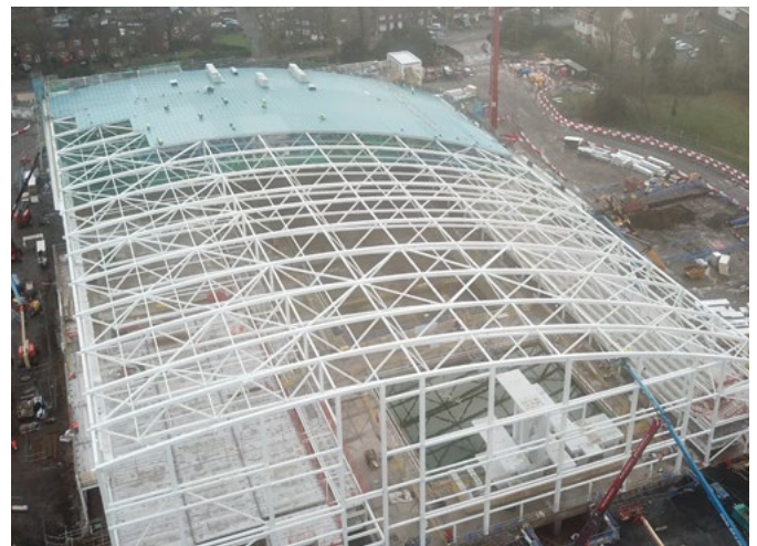
▶ Sandwell Aquatics Centre Construction
