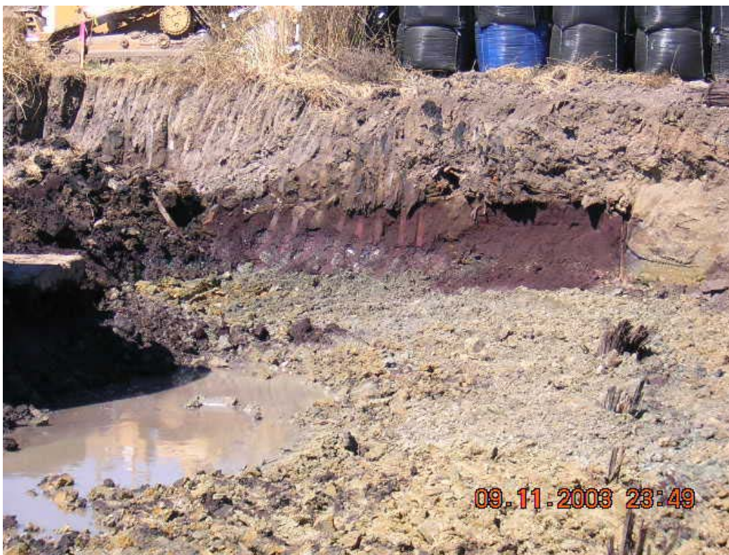
AREA 4 EXCAVATION (CINDER SOUTH OF SEAWALL)
