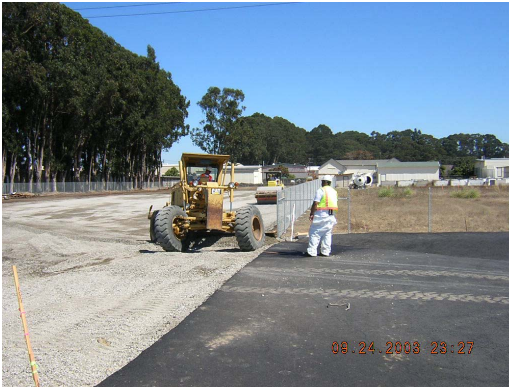
ASPHALT PAD CONSTRUCTION
