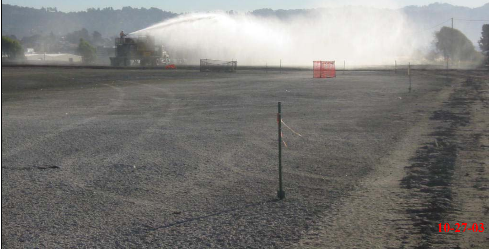
Spraying KUMA cap on top of treated Type A and B material on Zeneca property.
