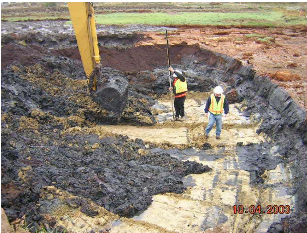
MARSH EXCAVATION BOTTOM
