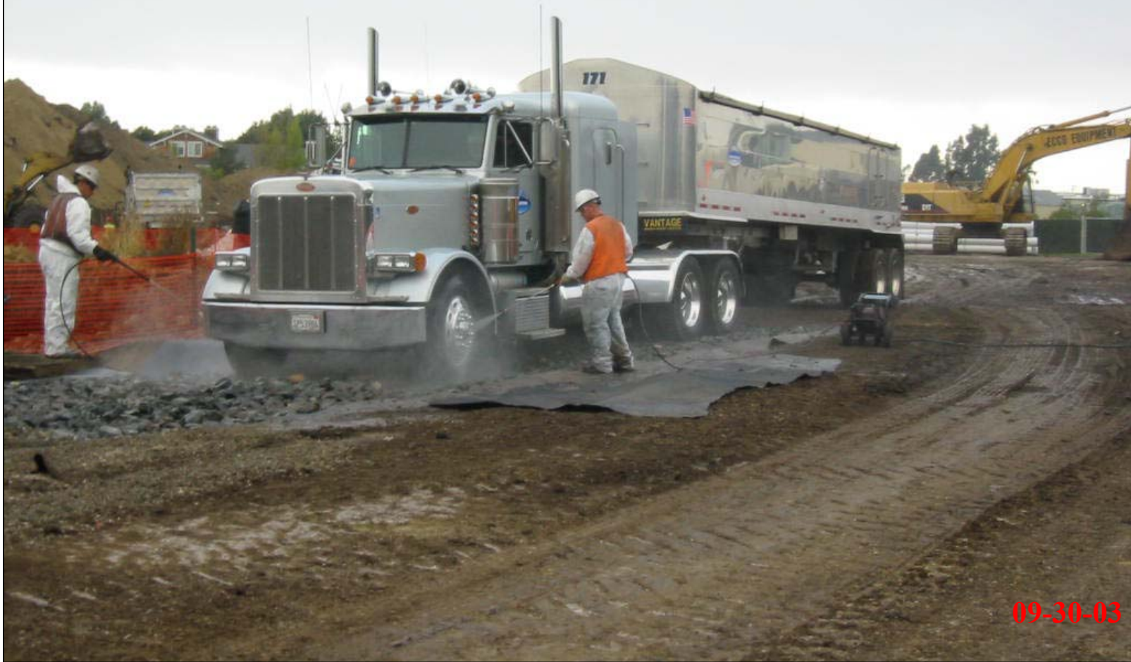
Pressure washing transport truck tires on decon pad prior to trucks leaving site for landfill.
