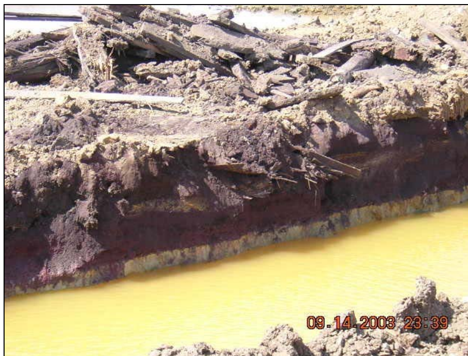
Figure 4. Wooden Box-flume continues into sidewall.
