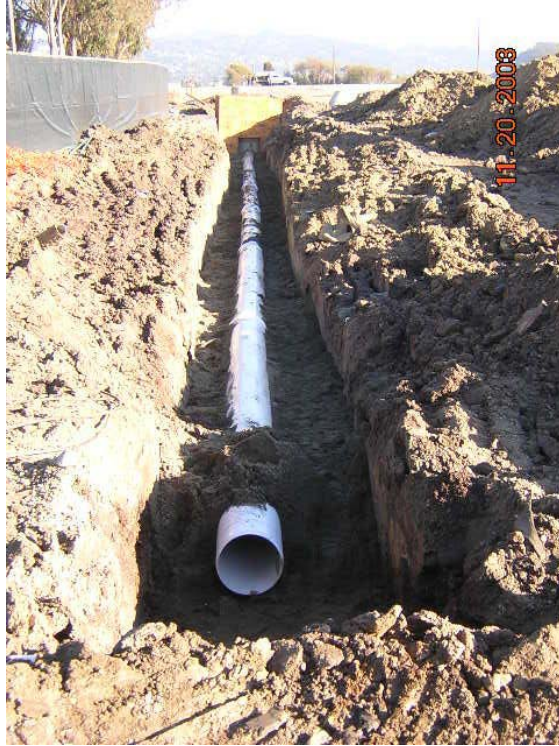
SANITARY SEWER INSTALLATION
