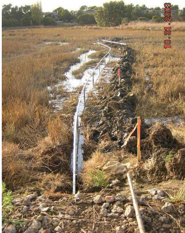
SILT SCREEN INSTALLATION
