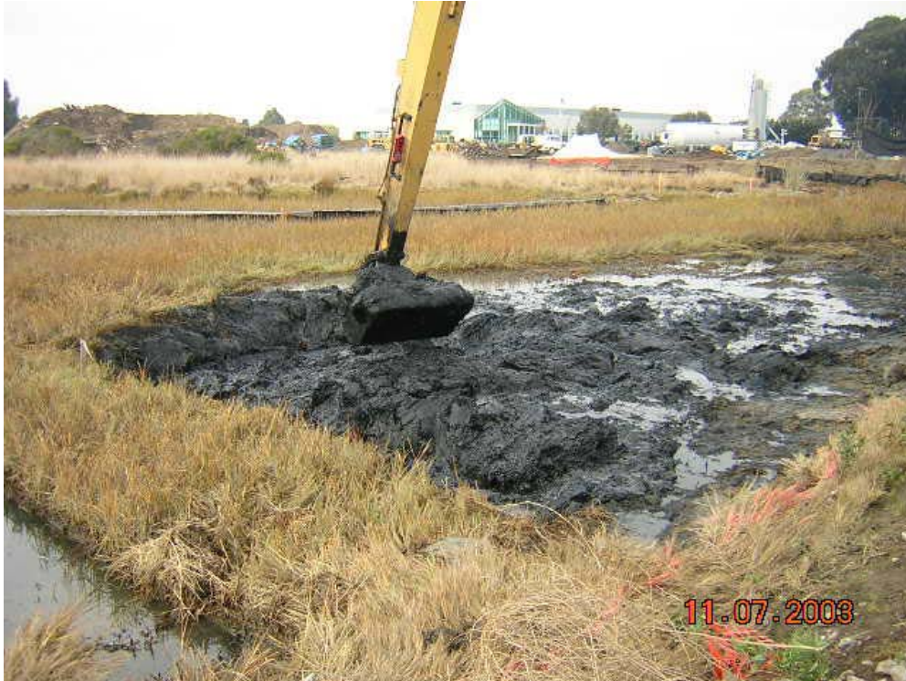
M3 MARSH EXCAVATION
