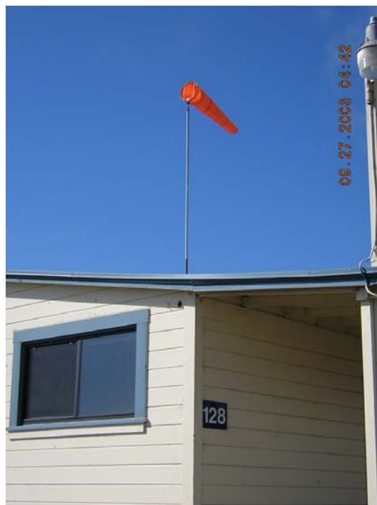
WIND DIRECTION MONITORING
