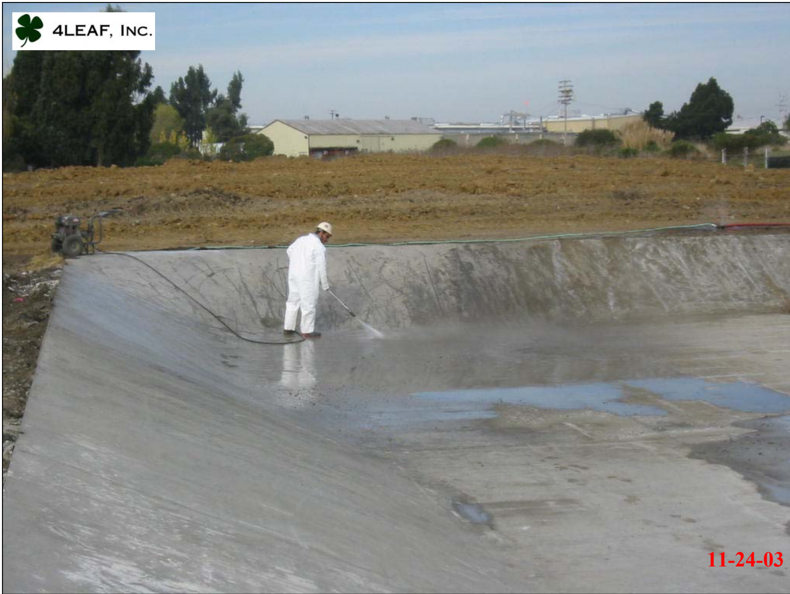
Using pressure washer to decon surface of concrete treatment pad after Type D soil was off loaded.
