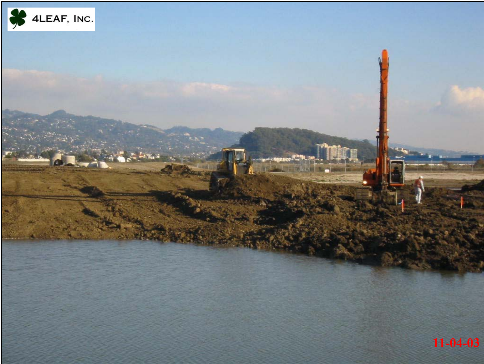
Backfilling Marsh Area 2 with clean Bay mud.
