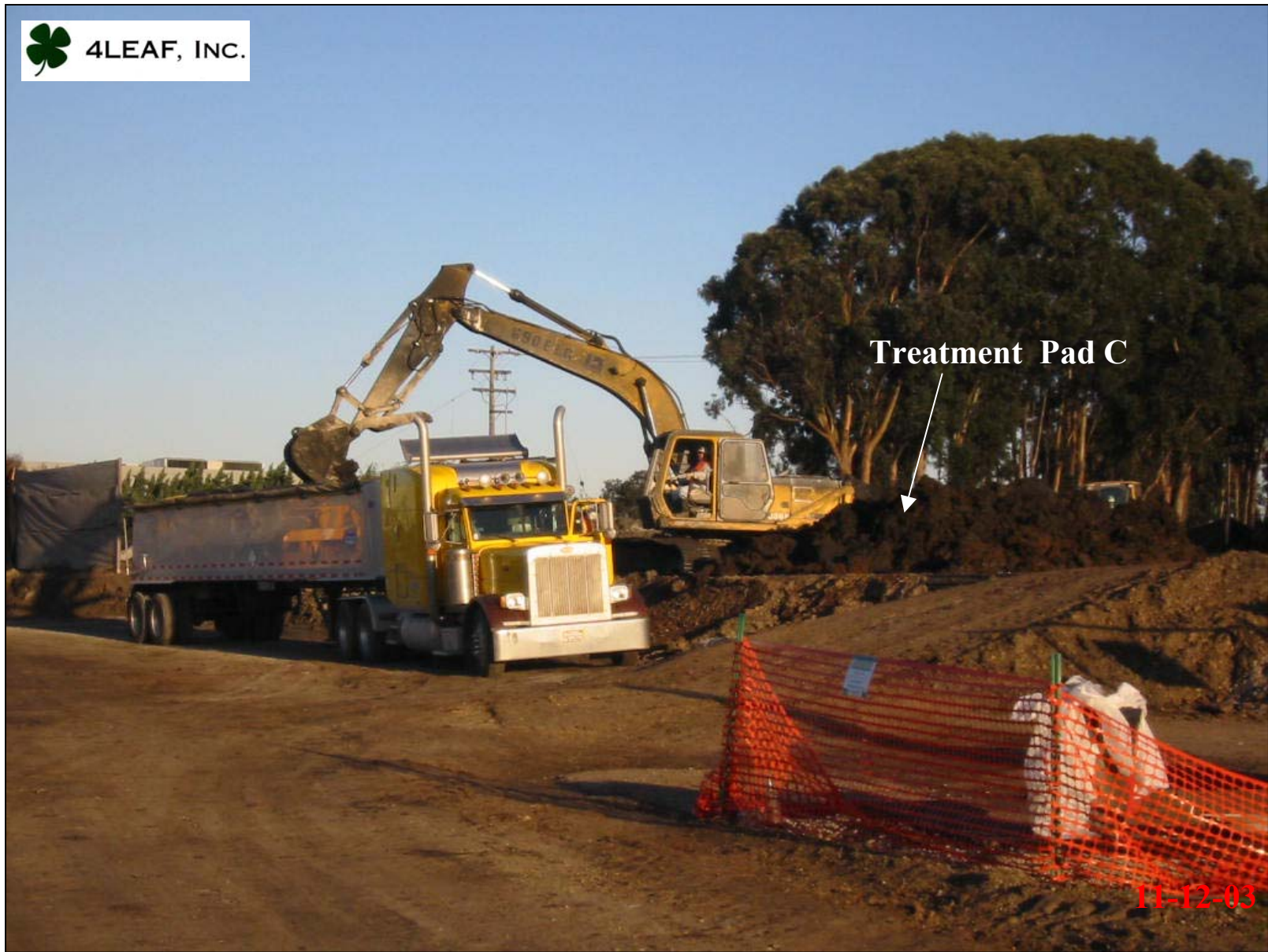
Loading mixed and dried Type C soil into off-site transport truck for shipment to landfill.
