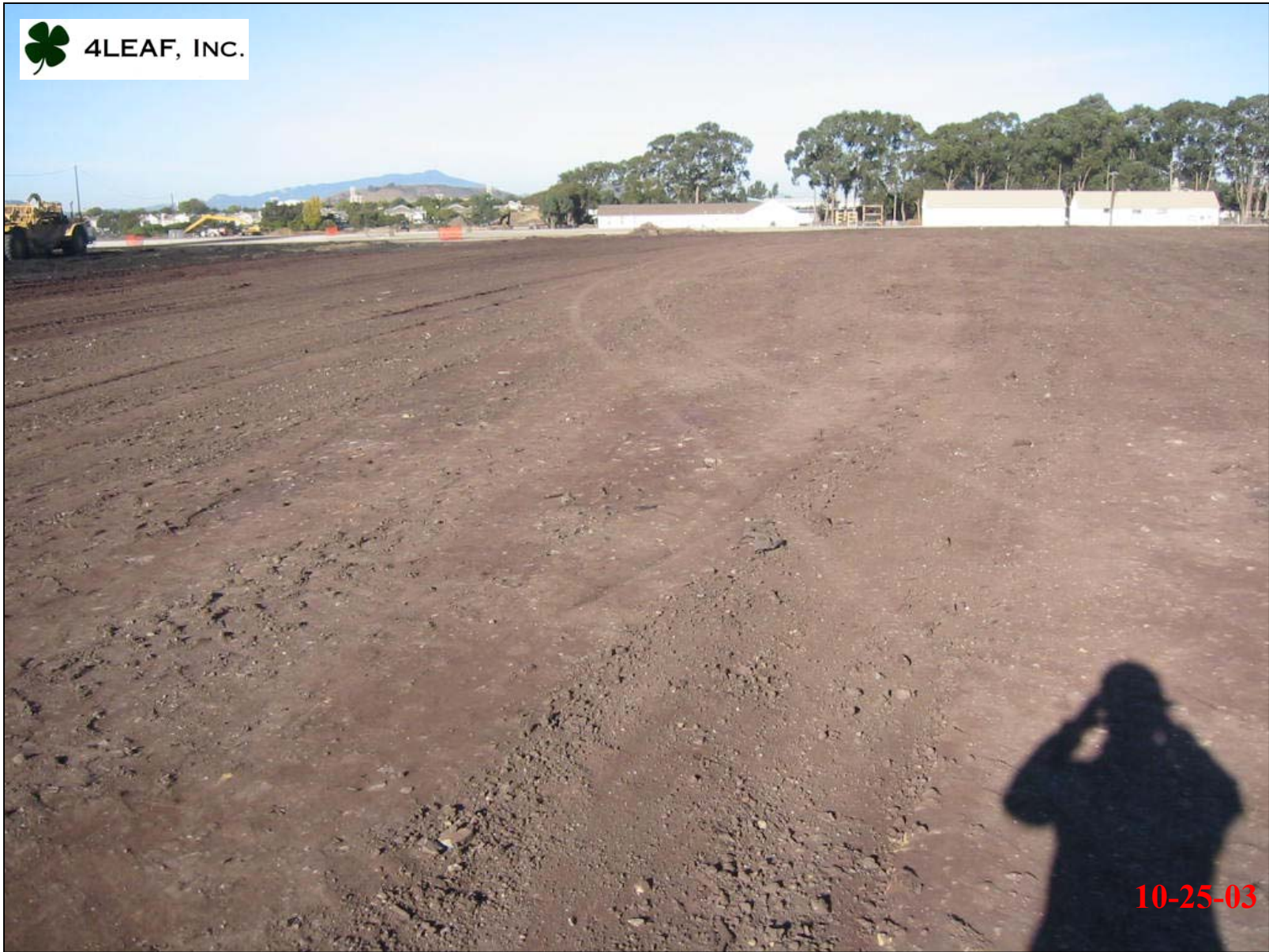
View of placed and compacted treated Type A and B material placed on Zeneca property.
