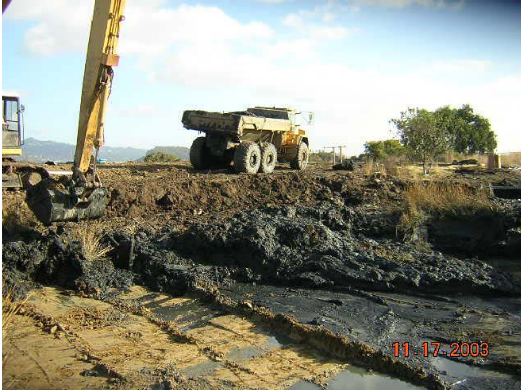
M1A MARSH EXCAVATION
