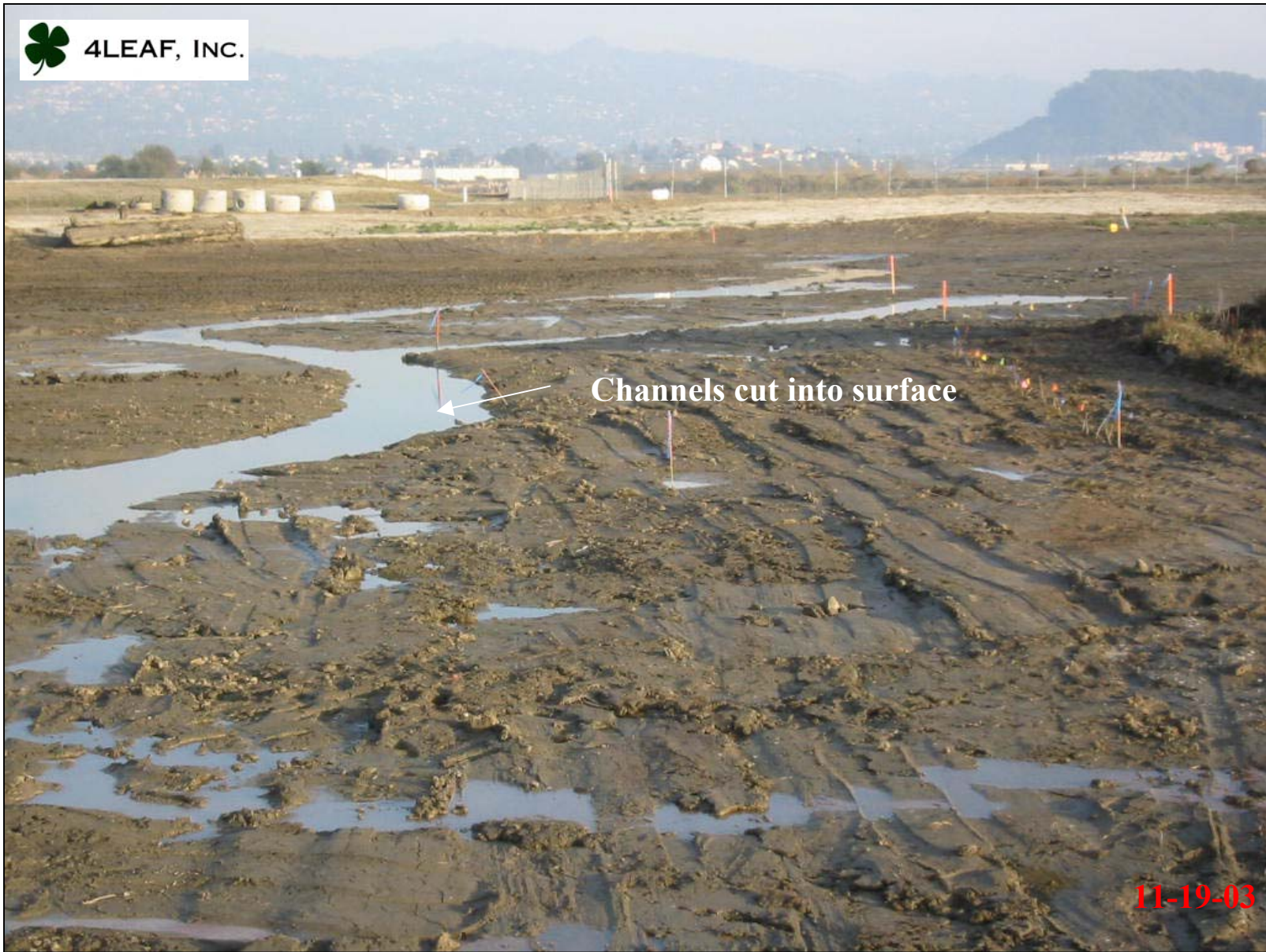
Regraded portion of marsh (excavated and backfilled during Y2002 activities).
