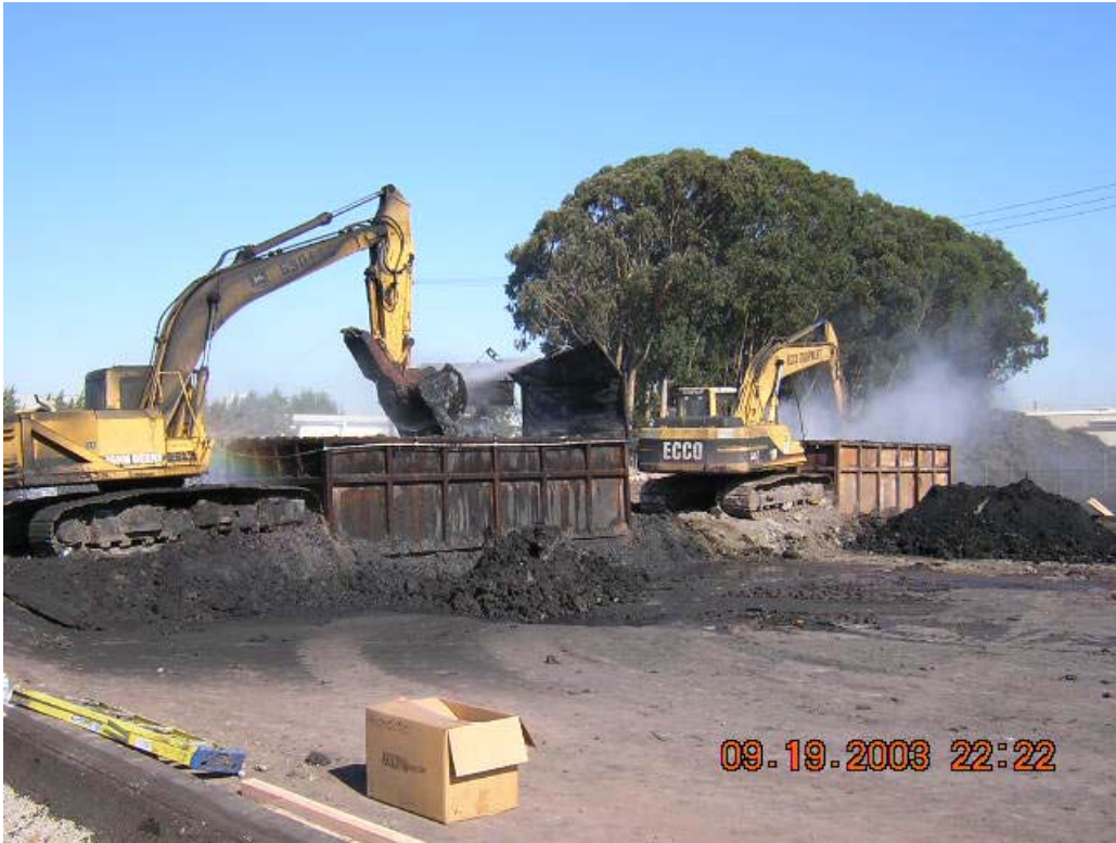
SOIL MIXING DUST CONTROL
