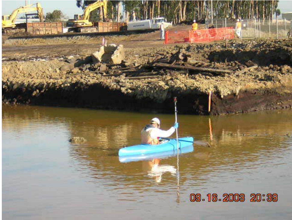
CONFIRMATION SURVEYING IN AREA 4
