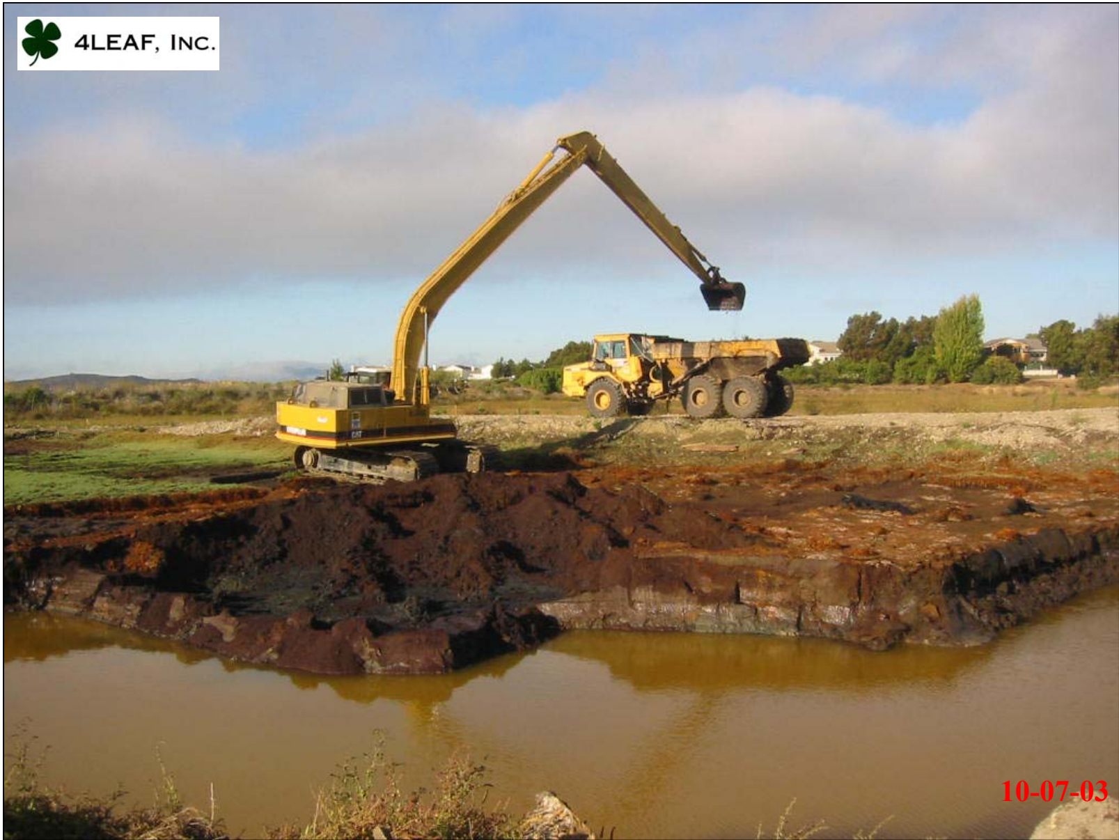
Excavating Type B soil from Marsh Area 2 (excavation area B-7).
