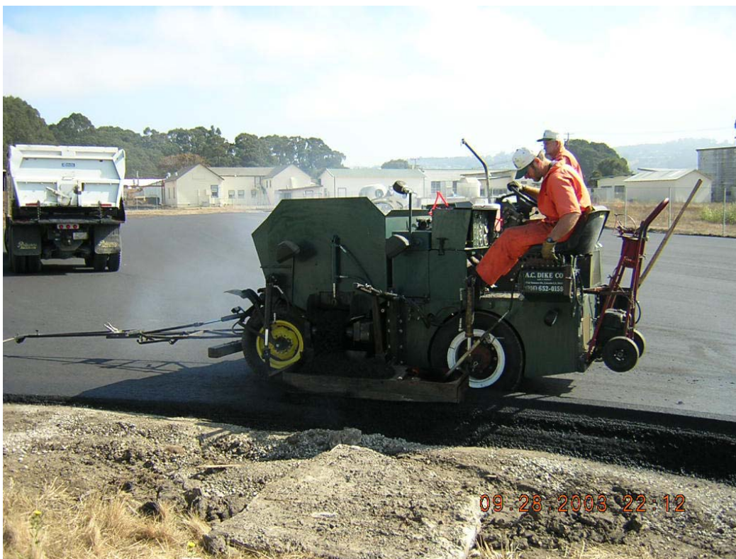
INSTALLING ASPHALT PAD BERMS
