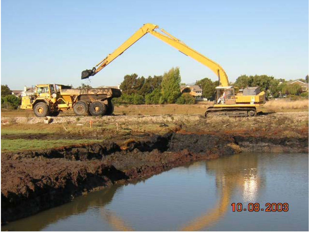
TRANSPORTING SEDIMENT TO TREATMENT PADS
