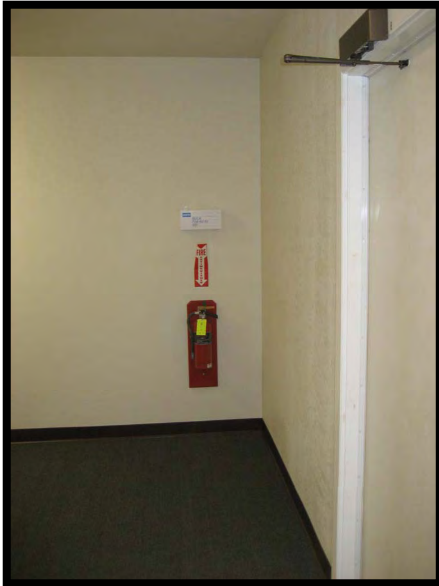
163-01, view of hallway
