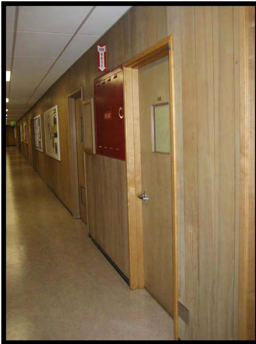
478-01, view of hallway outside office. New floor and ceiling tiles.
