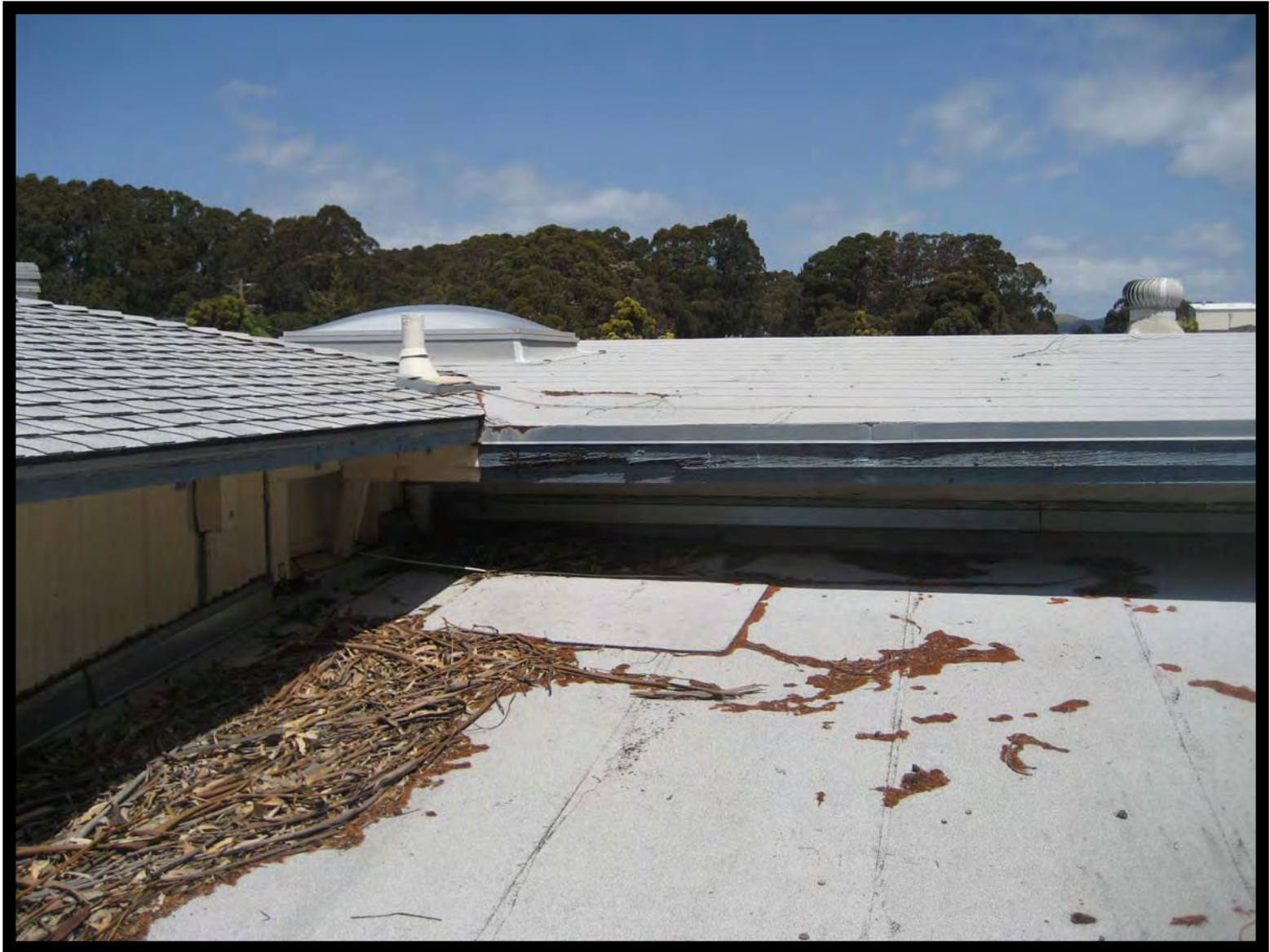
Sampling location 175-02. Sample was taken on upper part of the roof.
