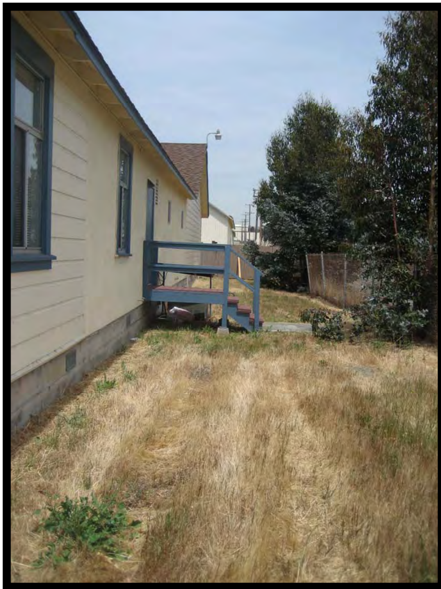
Sampling location 163-03. The sampling equipment was placed on the stairs.
