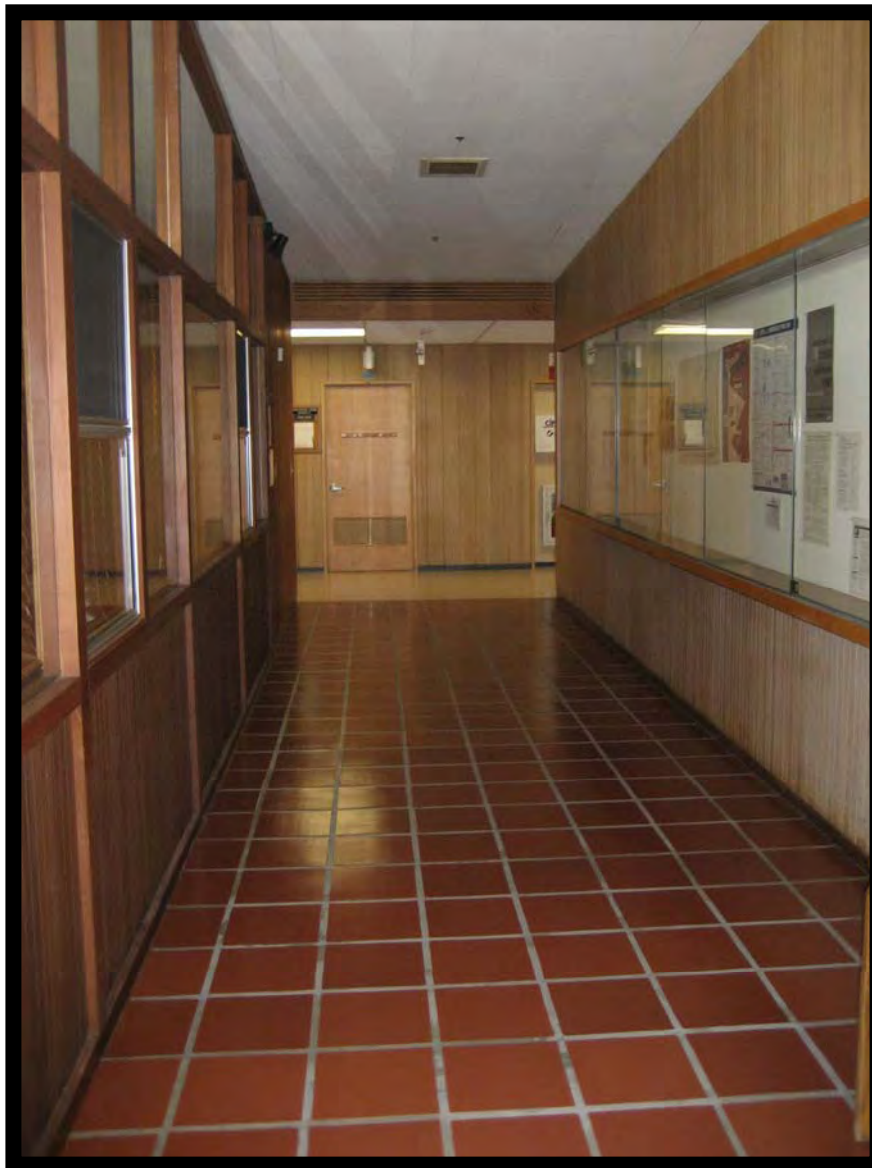
478-02, view from sampling location into adjacent hallway
