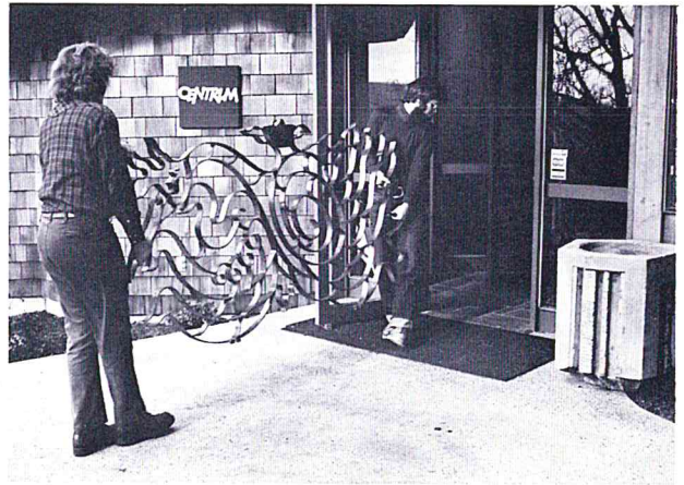
Keith Jellum (left) welded this steel gate in his studio and, with the help of Colin Page, installed it at the Oregon School of Arts and Crafts, where over twenty craftsmen were involved in producing elements of architectural detail. Works of two other craftsmen are shown here: a sign by calligrapher Tim Girvin and a cast concrete refuse container by Marge Hammond.
