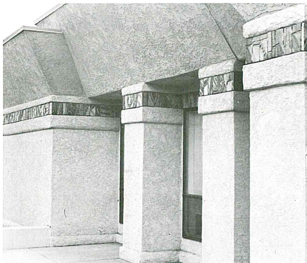
Ekos House. Williams was commissioned by the architects to design and manufacture a suitable decoration for the border of this entire building. The cost was established before work began. The tiles were placed in an existing groove.
