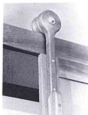
Detail of roller mechanism.
