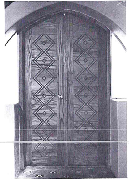
These doors in the same mosque were adapted from a traditional design in a book on Arab architecture written by the architect with whom Easton was working on this project.
