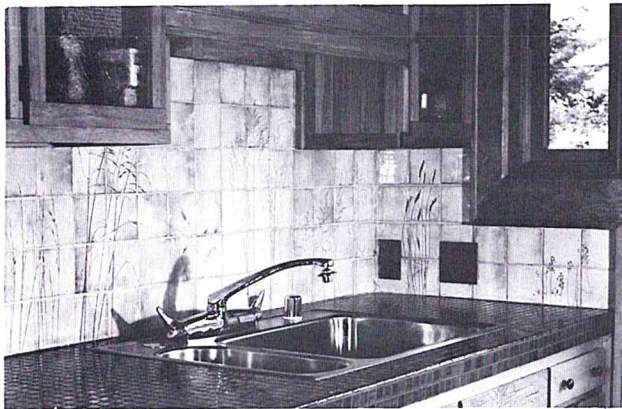
Waterproof sanitary wall surrounding kitchen sink area. Kluber reviewed his past work with the client, and a general design was agreed upon. Porcelain tiles with plants impressed into them were installed.
