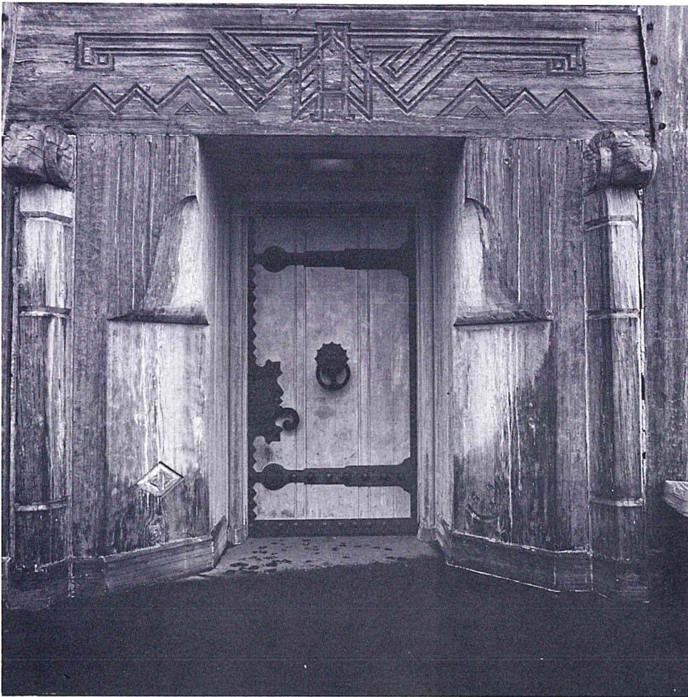
Main entrance to Timberline Lodge. The lodge was built and furnished by craftsmen working under the guidance of interior designer Margery Hoffman Smith, who was involved in the overall design and saw to it that patterns and designs were repeated throughout the building, both in furnishings and in structural elements.
