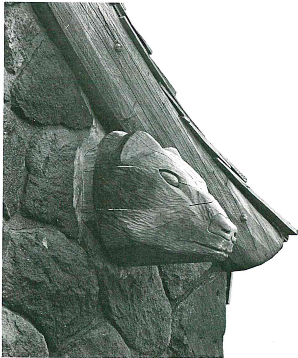
Carved wooden bear head on the end of a structural beam at Timberline Lodge.
