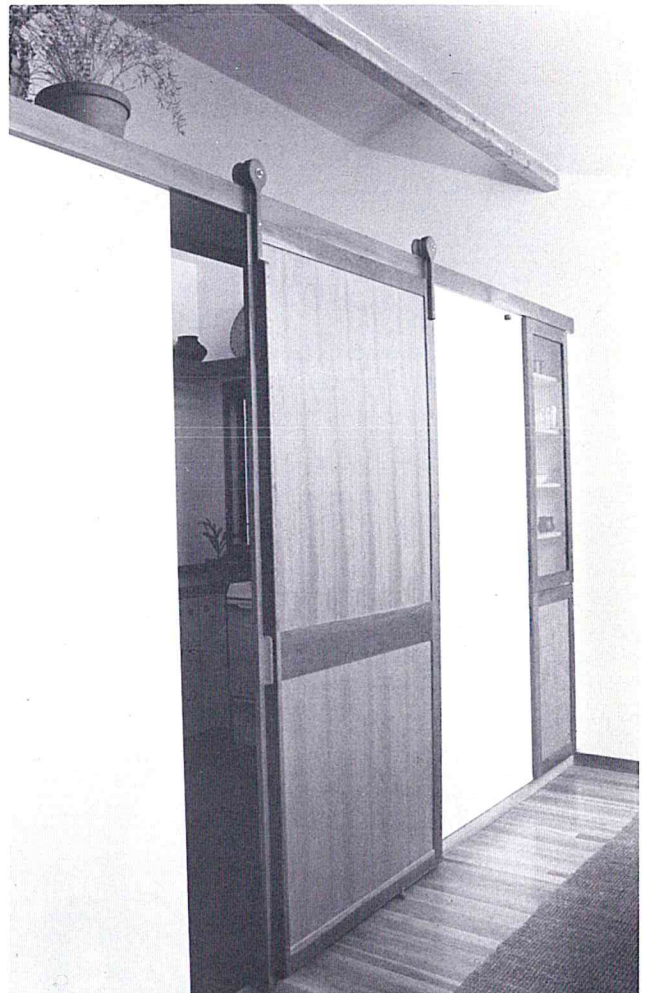
Sliding door and china cupboard. Von Rosenstiel designed and built the entire house. The client did not want to be cut off from guests while she was working in the kitchen, but she also didn't want the kitchen mess to be exposed to the guests' view. The sliding door and china cabinet (which do not go to the ceiling) allow the openness she wanted, but the door can be closed to hide the food-preparation disorder. The china cupboard opens on both sides.
