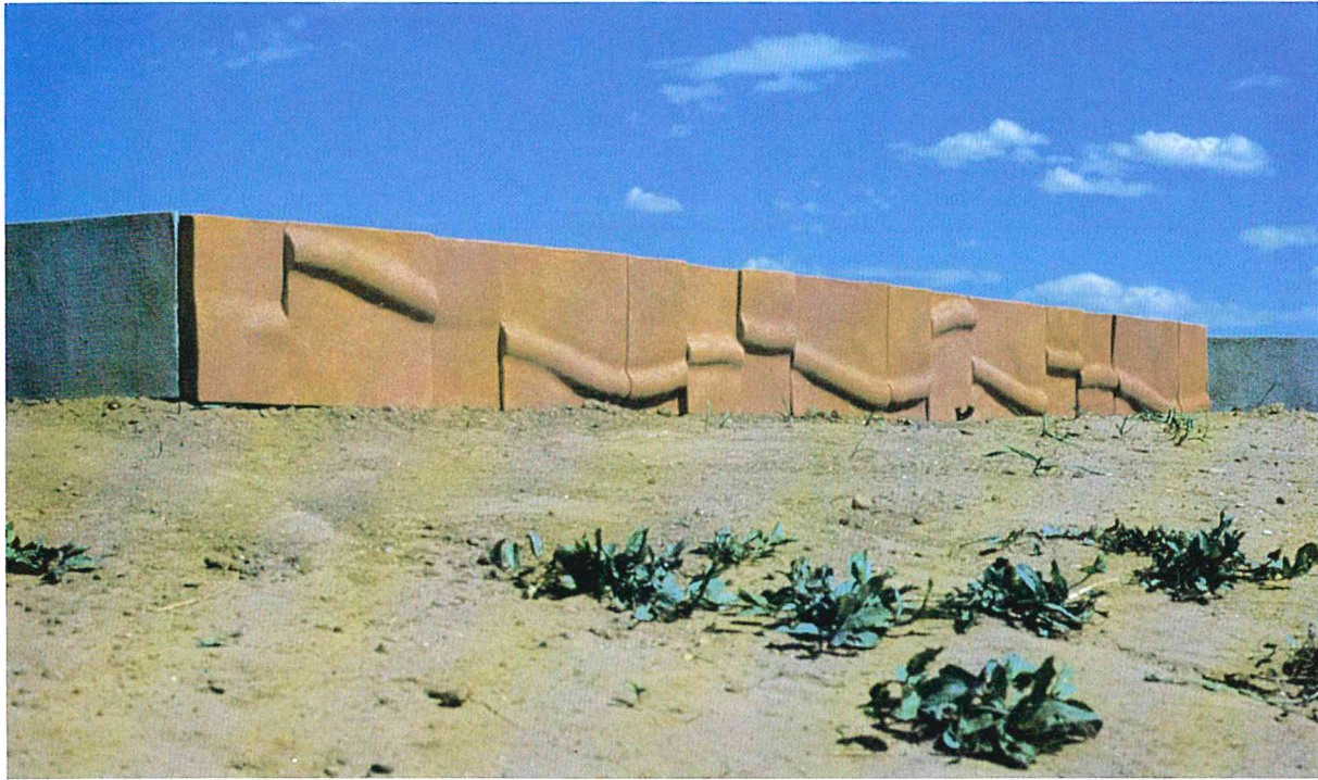
Sandra Robishaw constructed Fiberglas molds for the concrete contractor to use
