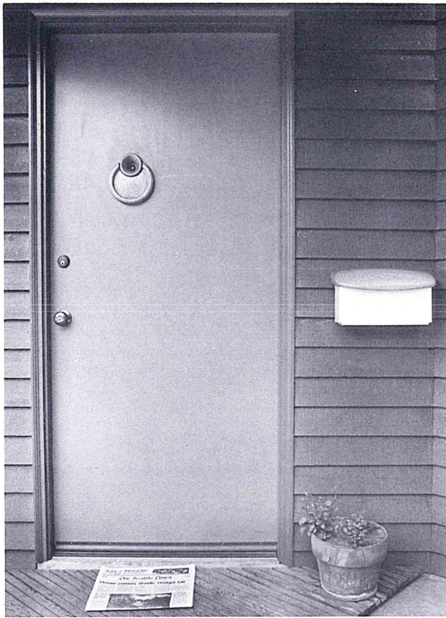
Door knocker and security peephole. Von Rosenstiel incorporated both functions into one object. When the wood plug is removed from the door knocker, it is possible to see who is at the door.
