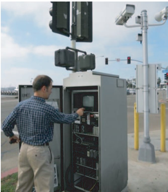
Figure H-20. Jon Hannasch conducts a system check on a red light camera system.
