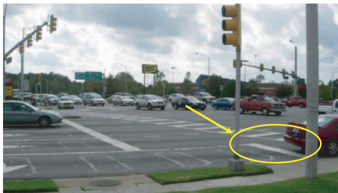
Figure H-11. Location where right turn lane stop bar was relocated after observing a high number of false violations during the warning period.
