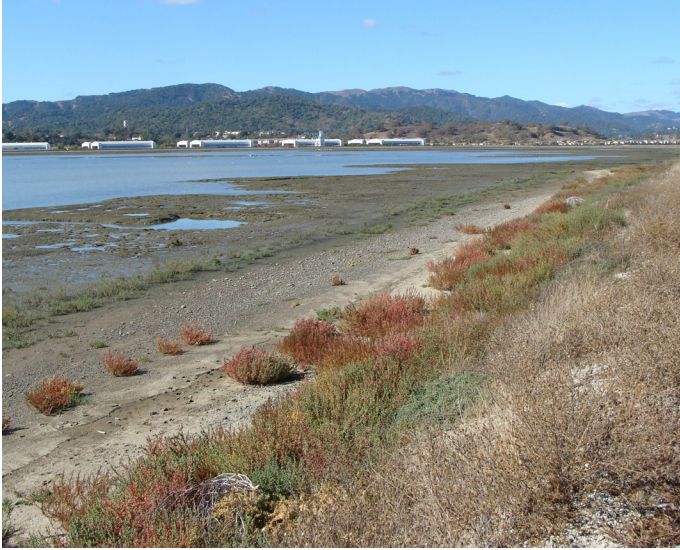
▲ Figure 29: The habitat-friendly levee bench on the north side of the project after 1.5 years has vegetated and resisted erosion although it has settled more than expected and may require additional sediment placement. Photo credit: Damien Kunz.
