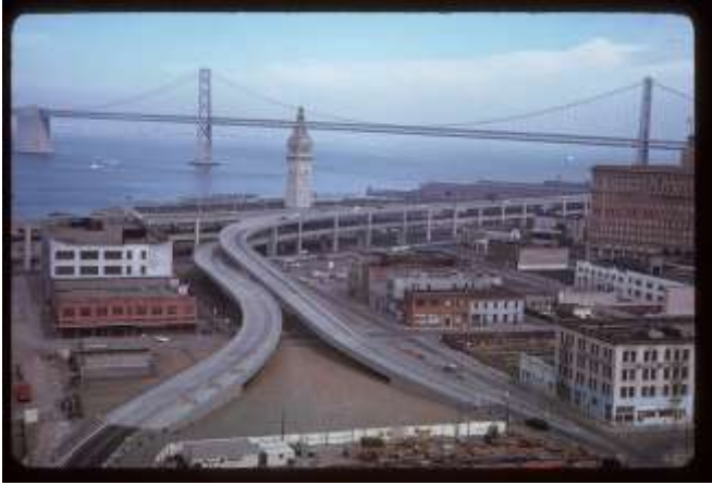
Figure 6.4: Embarcadero Freeway ending at the Broadway off-ramp (Lost SF, 2010)
