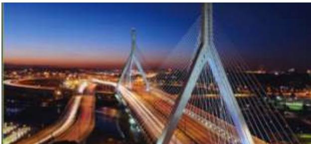
Figure 1.1: The Zakim Hill Bridge
