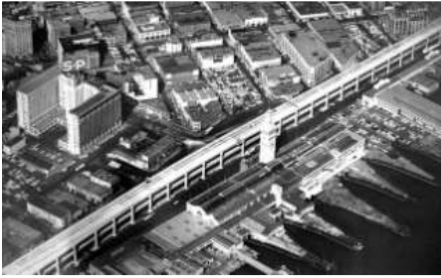
Figure 6.5: Embarcadero Freeway, 1960. (Source: Telstar Logistics)
