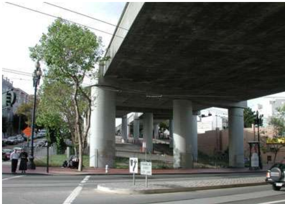
Figure 5.2: The southern portion of the Central Freeway loomed over Octavia Street.
