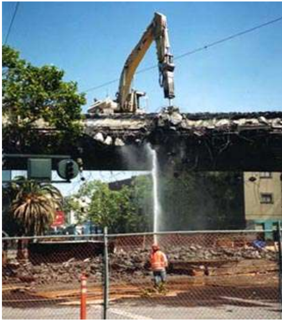
Figure 5.3: Demolishing San Francisco's Central Freeway (Preservation Institute, 2007)
