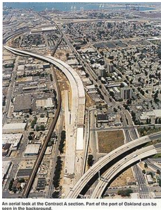
Figure 2.3: Cypress Freeway. Source: Federal Highway Administration
