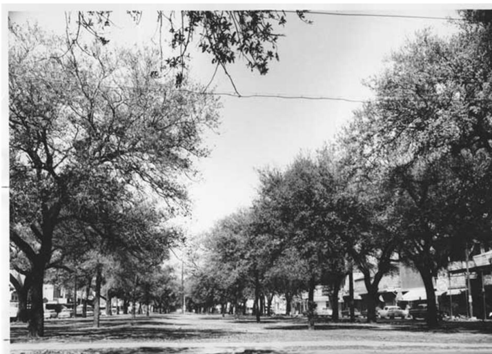
Figure 3.1: North Claiborne Avenue, at Dumaine Street, looking towards Elysian Fields. "Oak Tree Conservation." Undated. City Archives New Orleans Public Library
