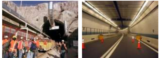
Figure 1.2: Construction of the Tunnel
