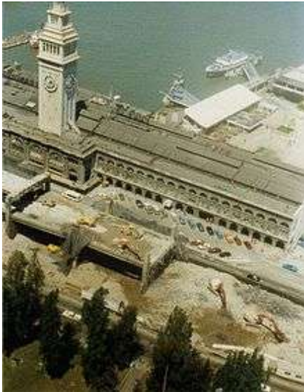
Figure 6.3: Embarcadero Freeway Demolition. May 9, 1991
