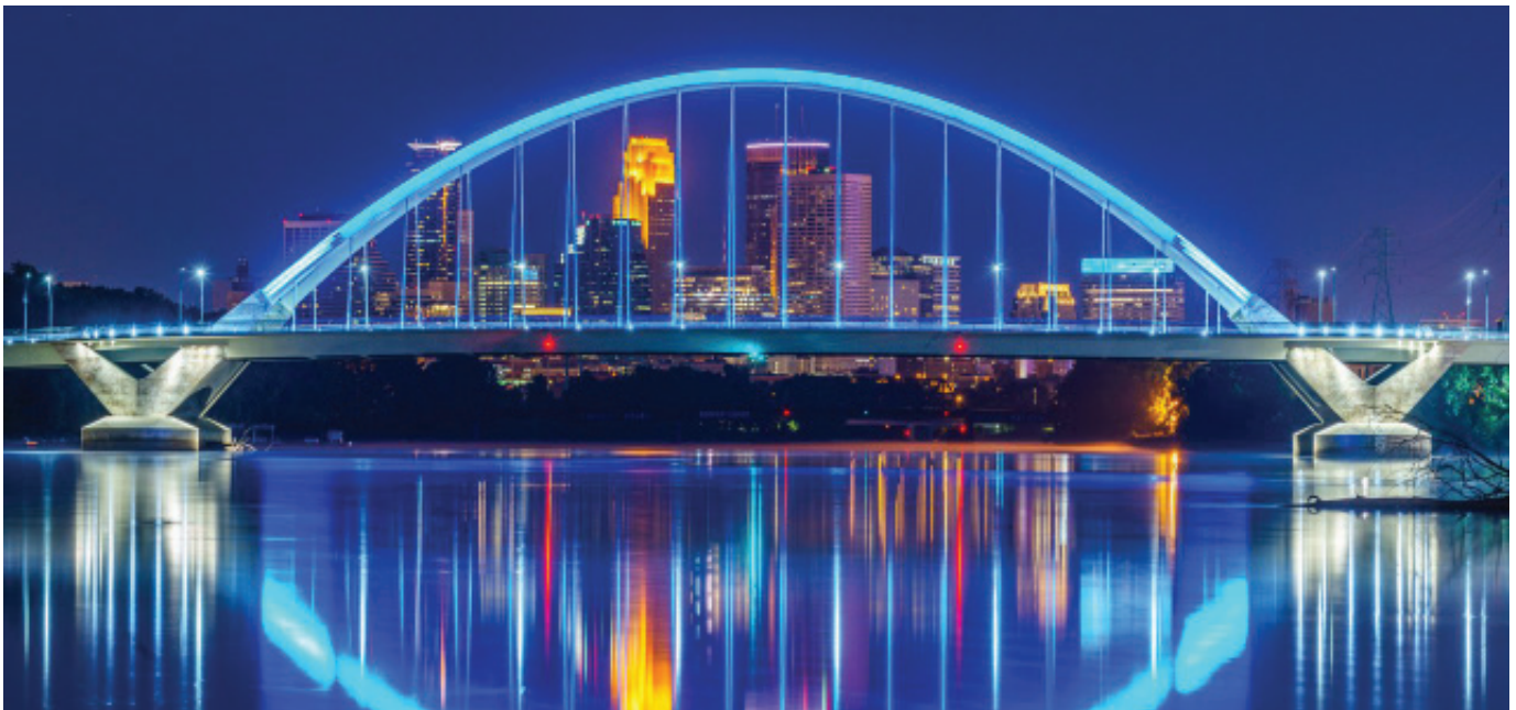
Lowry Avenue Bridge / Courtesy of Meet Minneapolis
