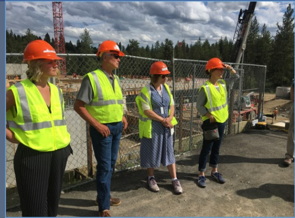
Tour of the Next Level Treatment under construction at the Riverside Park Water Reclamation Facility in Sept 2019. Photo Credit: Hannahlee Allers
