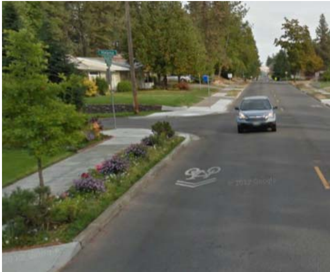
Figure 3. Examples of Shared Roadway treatments
