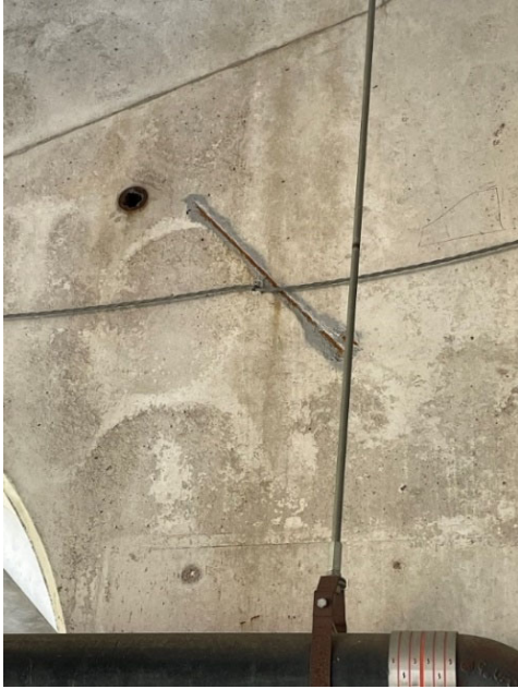
Figure S-2: Exposed Reinforcement Location: Typical Outdoor Seating
