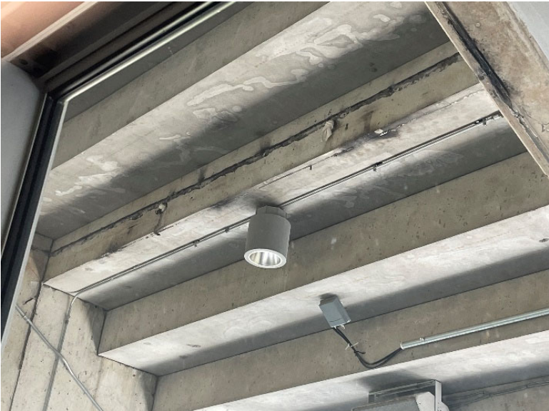
Figure E-4: Beneath Grandstands Location: Loge Level Suite
