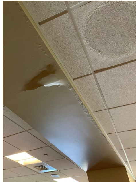
Figure AI-5: Water Damage Location: Various Concession Stands
