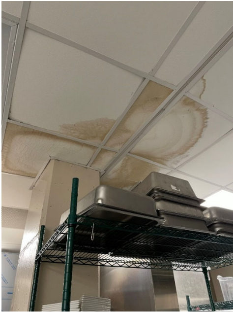
Figure AI-5: Water Damage Location: Various Concession Stands
