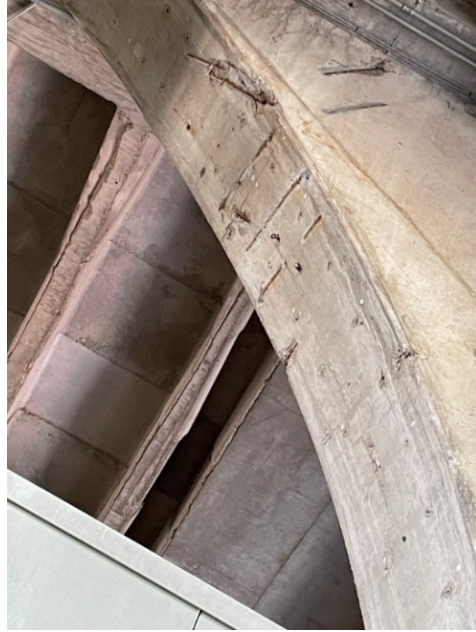
Figure S-2: Exposed Reinforcement Location: Typical Outdoor Seating
