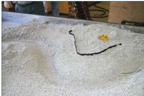
Installing a silt fence.
