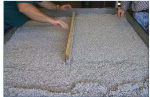
Smooth out the grit with a leveling board.
