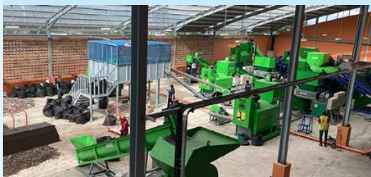
FIGURE 5. New integrated solid waste treatment facility that has been constructed and is in preparation for operation in Cimahi City, Indonesia. Photo credits: Aulia Syahrani.
