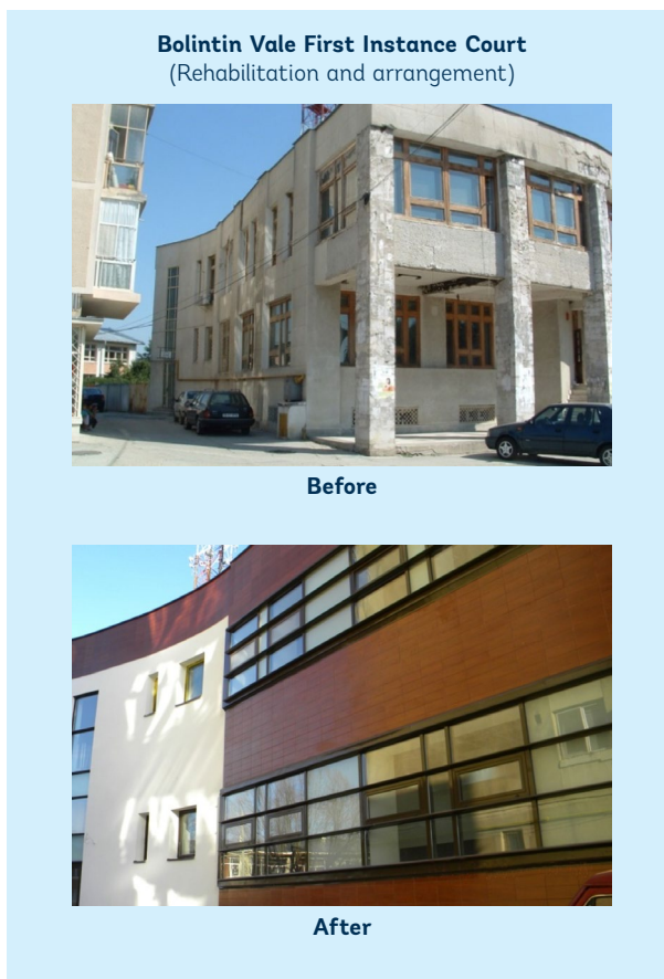
FIGURE 9. Examples of recent investments in justice infrastructure
