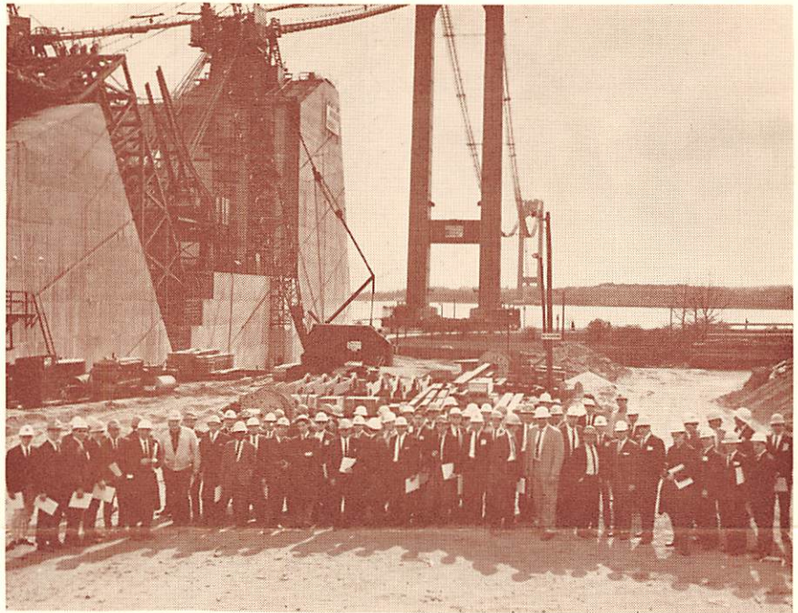
HARD-HATTED engineering students from 20 colleges are shown against impressive backdrop of Verrazano-Narrows Bridge, a feature stop on the big Students' Day staged by The Moles as part of its educational program, last April 26. Other stops were the new Flushing Stadium, and various buildings of the burgeoning 1964 World's Fair.
