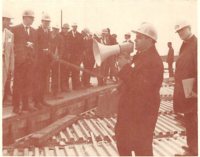
Nick Cifelli, Highway Engineer (construction) New Jersey Dept. of Transportation, explains bridge deck construction over the Penn Central RR Waverly Yards for the interchange complex of Route 78, to a group of students at The Moles' Students' Day Field Trip April 5.
