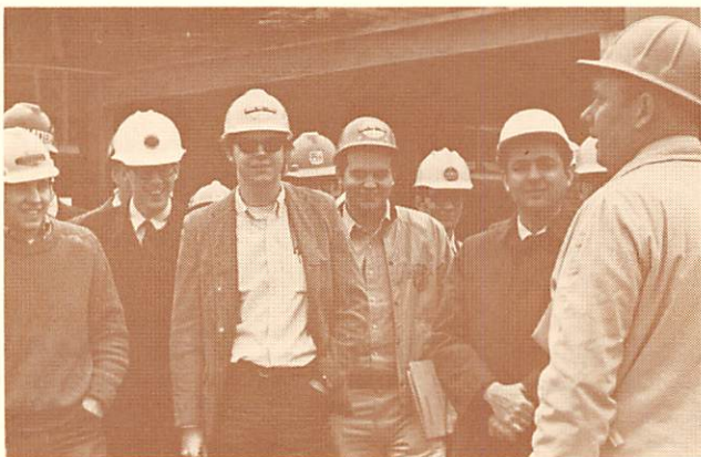
The steel frame goes up in a hurry but then begins the interior finishing. . . .
