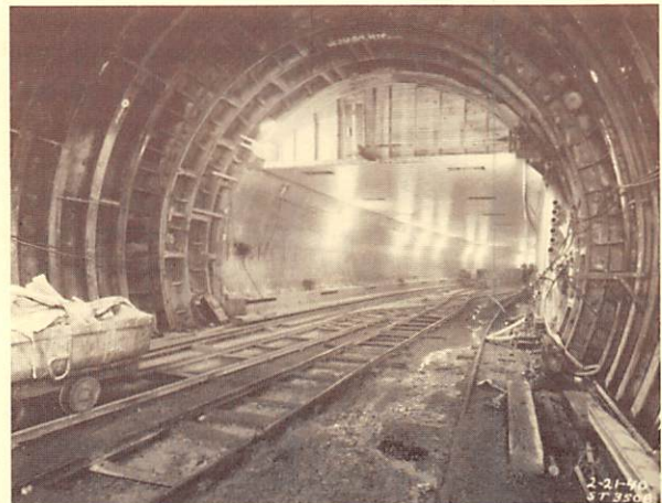
Cast iron tunnel lining with concrete lined tunnel in background - 2/21/40.
