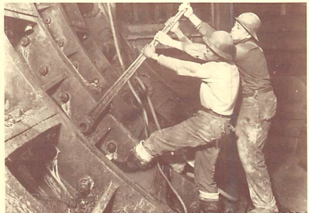
Sand Hogs tightening a bolt in cast iron lining with 5 foot ratchet wrench - 2/26/39.
