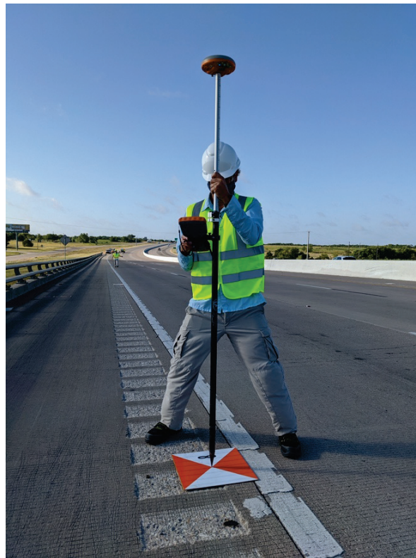
Figure 181. RTK Surveying of Targets.
