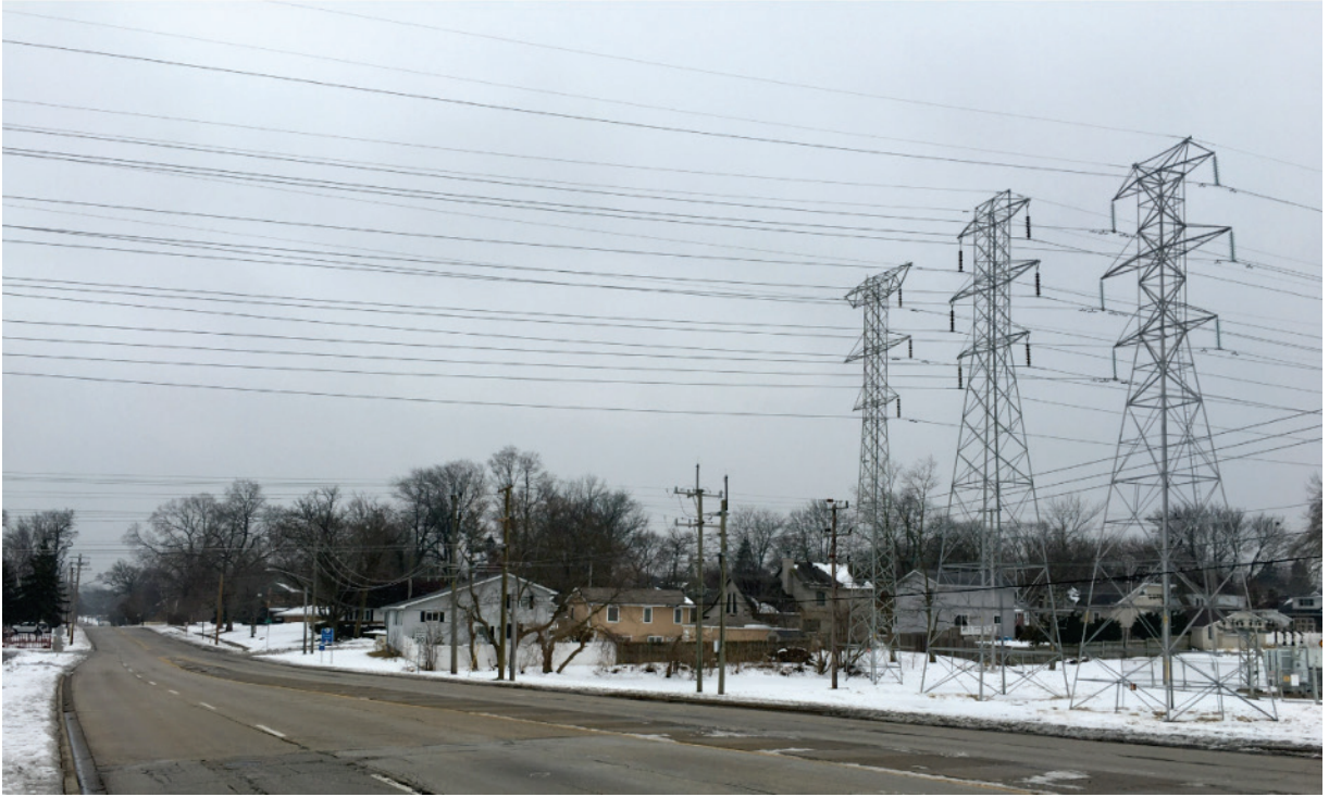
Figure 20. Electric Transmission Towers in Waukegan, Illinois.
