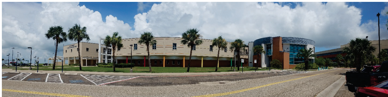
Figure 137. ECDC Building on the TAMUCC Campus.
