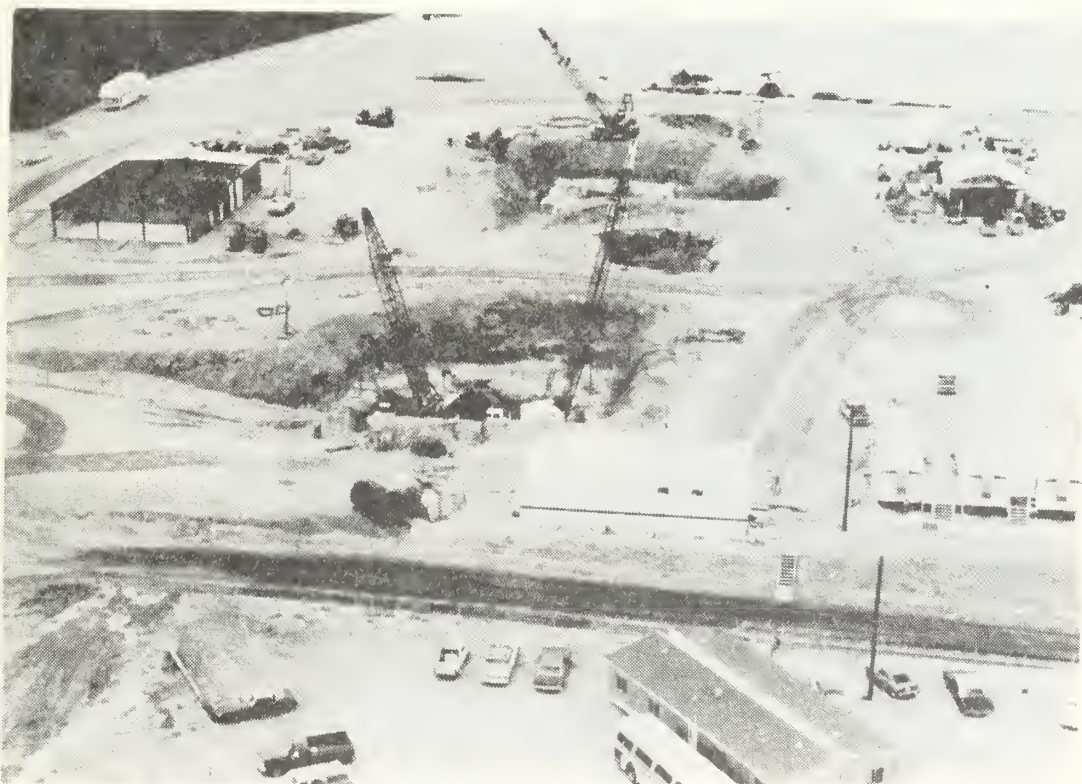
Construction progress in the Mine Support Area
