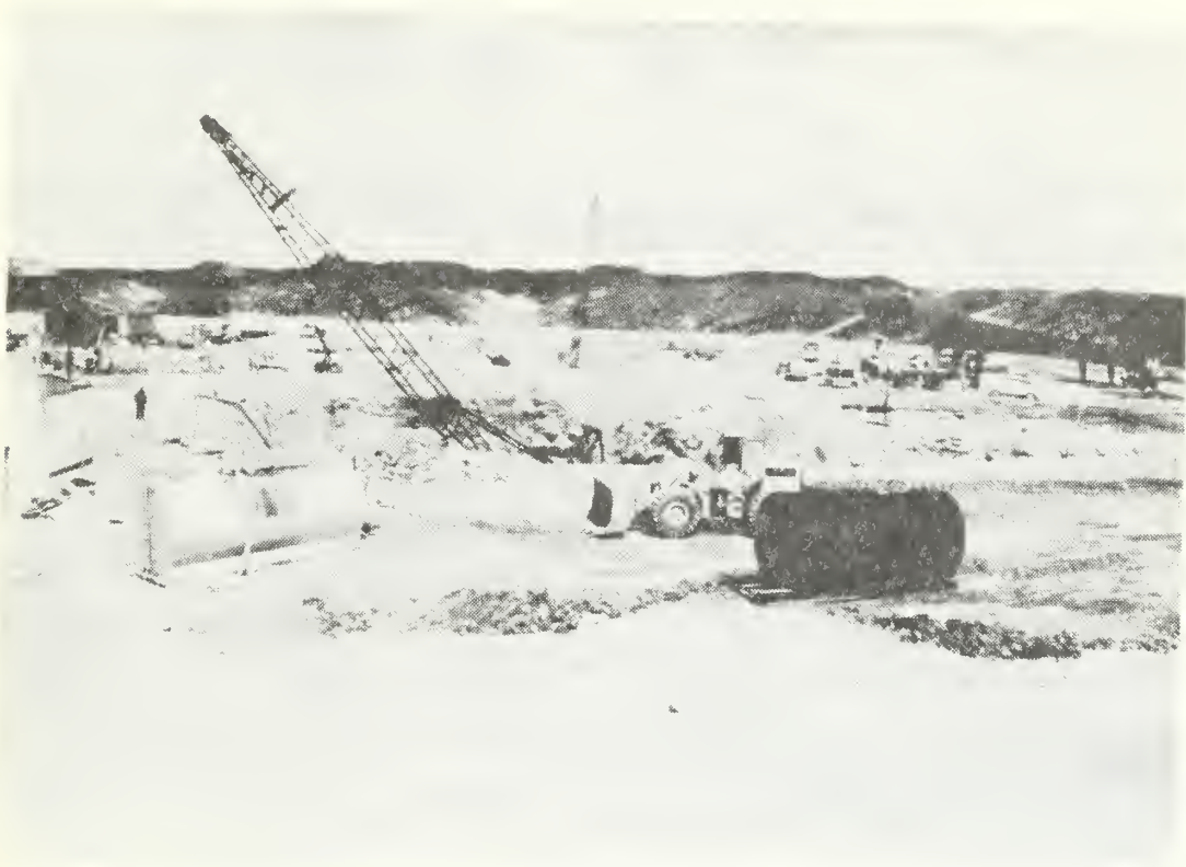
Shaft collar and foundation excavation in the Mine Support Area and erection of temporary Maintenance Building
