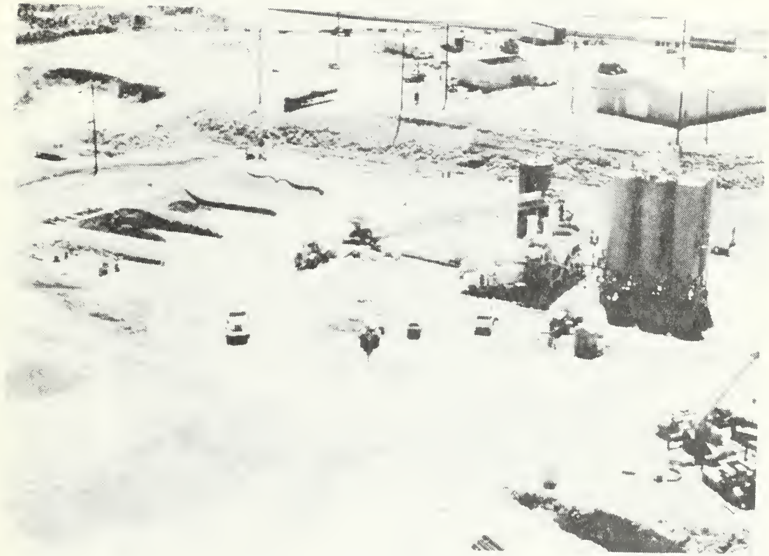
Operational Concrete Batch Plant
