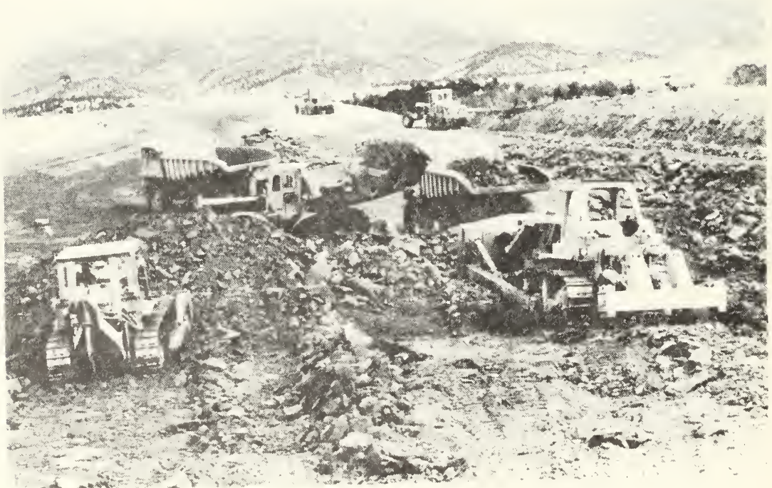
Earthwork - Cut-and-fill activities in the Mine Support Area
