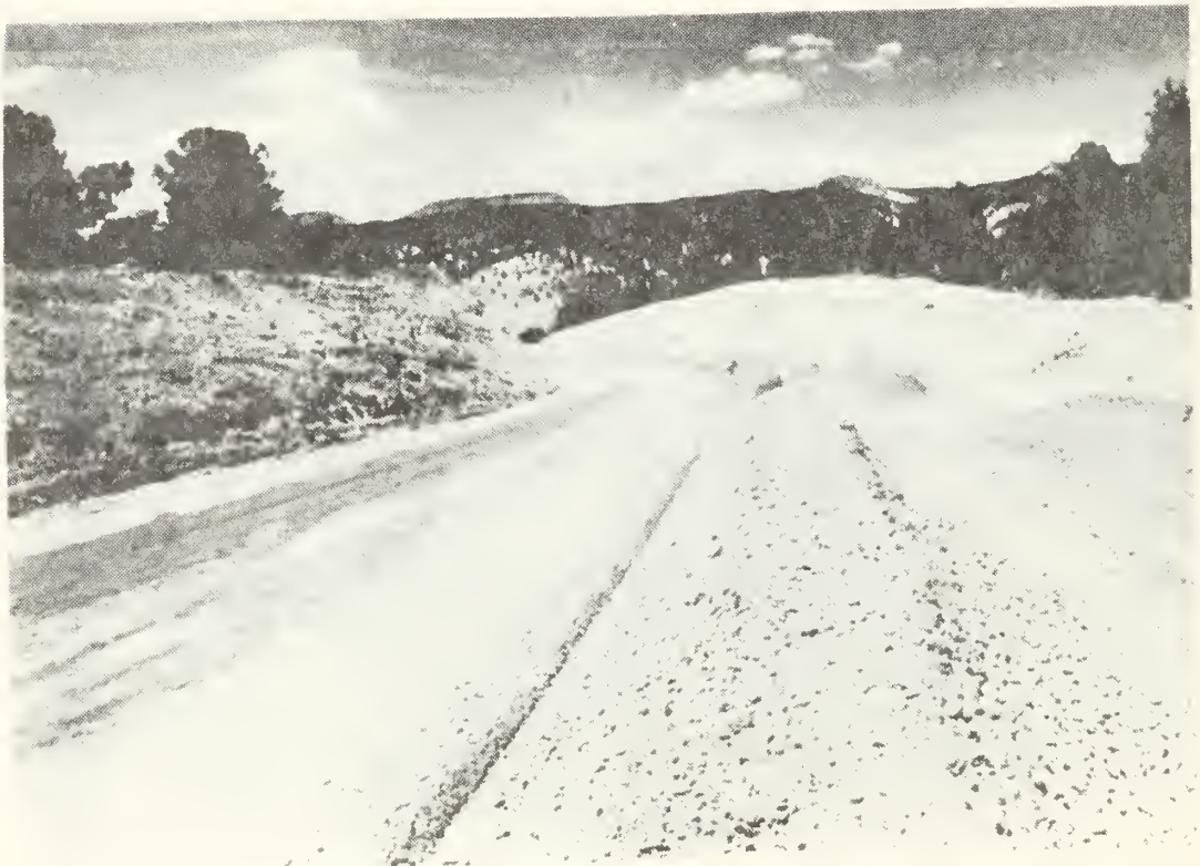
Final touches on the road surface
