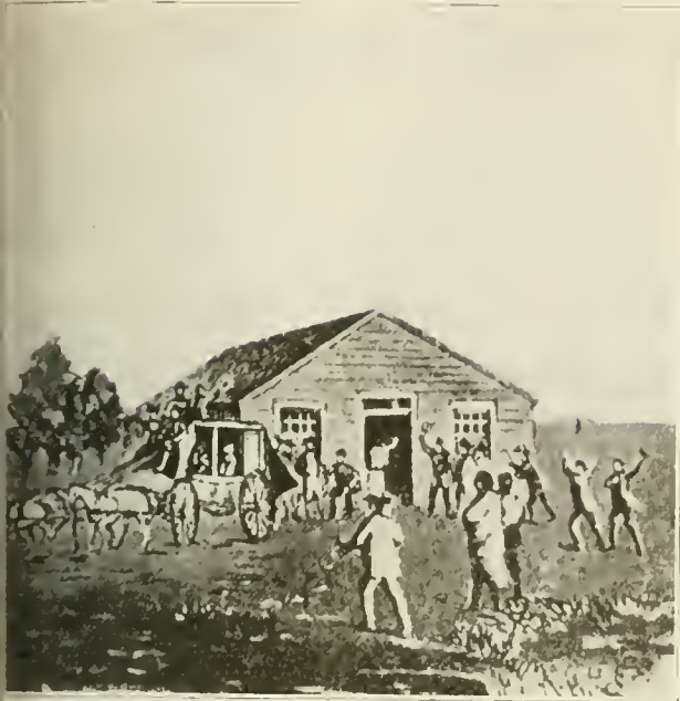
Office of the Leavenworth & Pike's Peak Express Company, built in the autumn of 1859. This company operated the first line of stage coaches into Denver, which was also the first into the Pike's Peak gold country.
