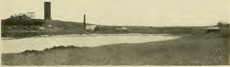
Standpipe—Wannacomet Water Works
