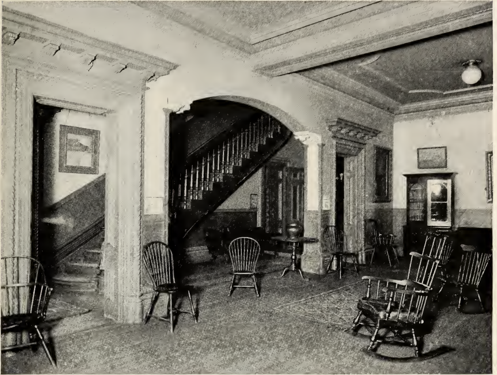
Reception Hall — Hull-House
