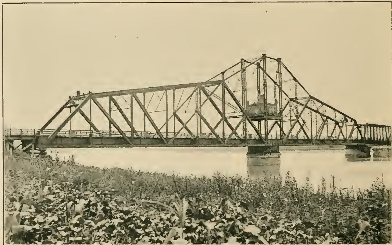
ILLINOIS CENTRAL RAILWAY BRIDGE OVER MISSOURI RIVER LONGEST DRAW SPAN IN THE WORLD
