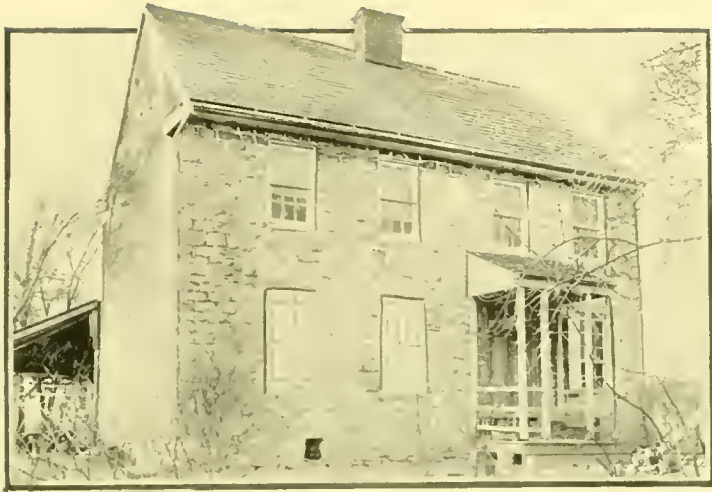
THE COOKES HOUSE ON KING'S MILL ROAD, WHERE THE GOVERNMENT RECORDS WERE FIRST DEPOSITED ON SEPTEMBER 30, 1777
