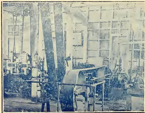
MECHANICAL ROOM, ALABAMA POLYTECHNIC INSTITUTE.
