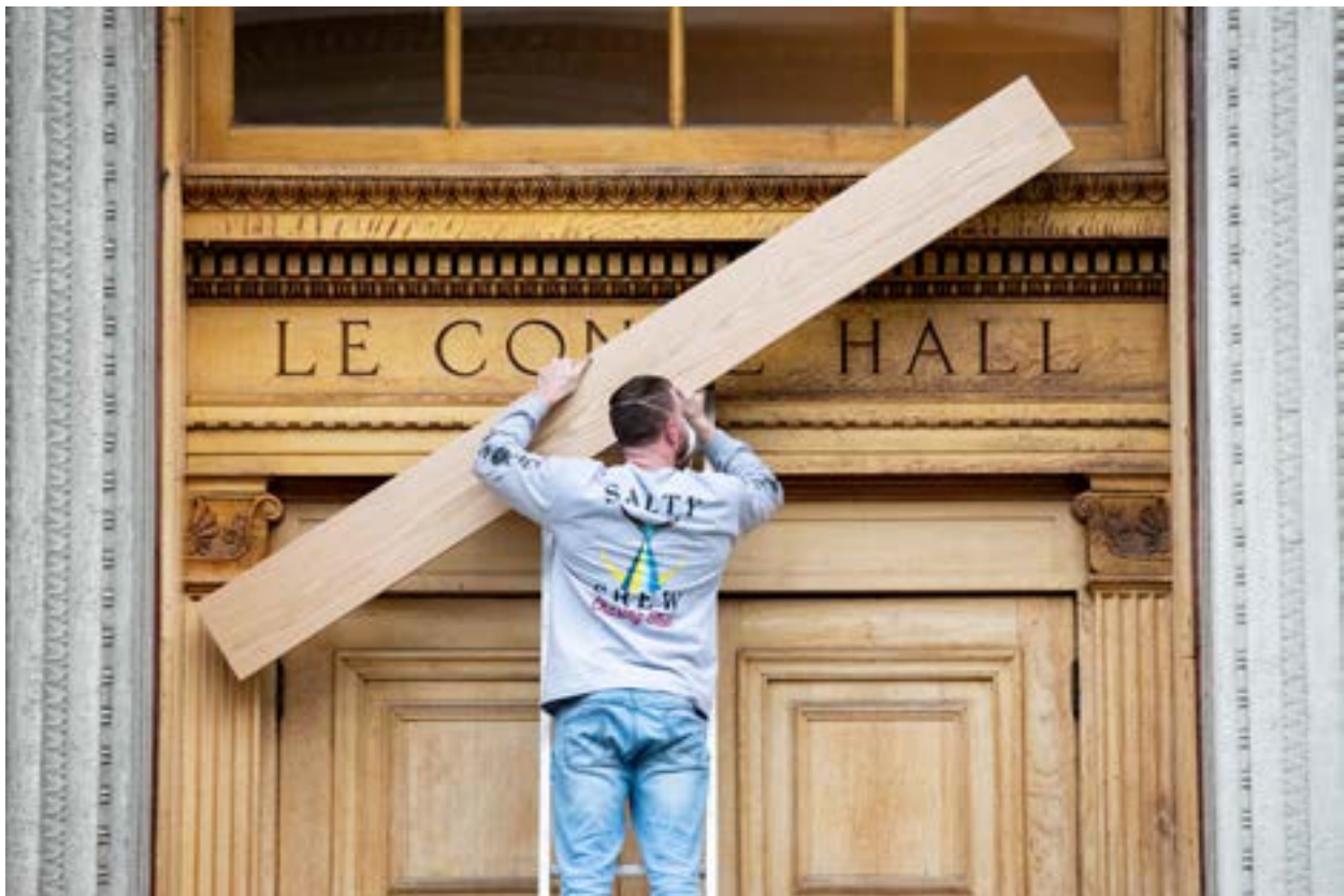
Joseph Poppi of Facilities Services installing oak panels as part of denaming LeConte Hall, November 2020. Photo: Irene Yi.
