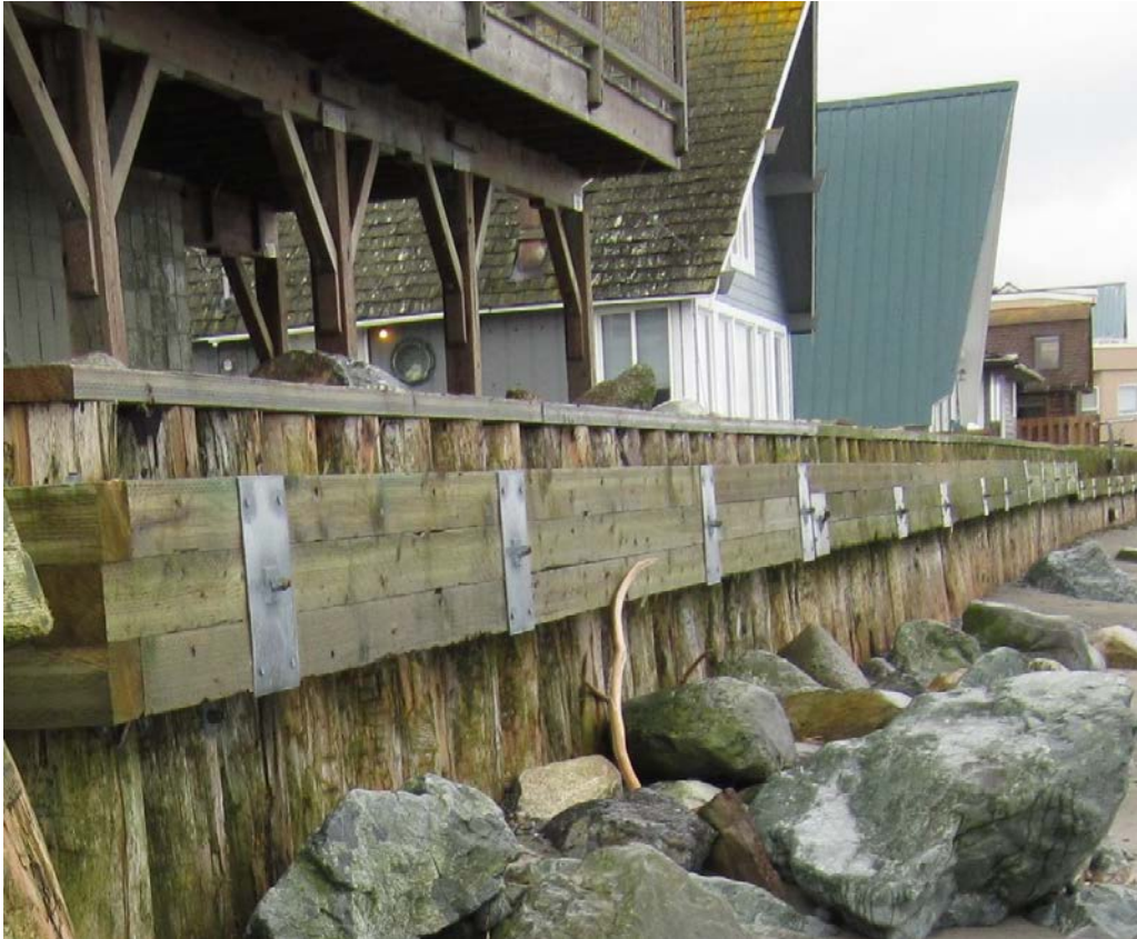
Figure 7.5-13. Armor stone toe protection at a Puget Sound vertical bulkhead.
