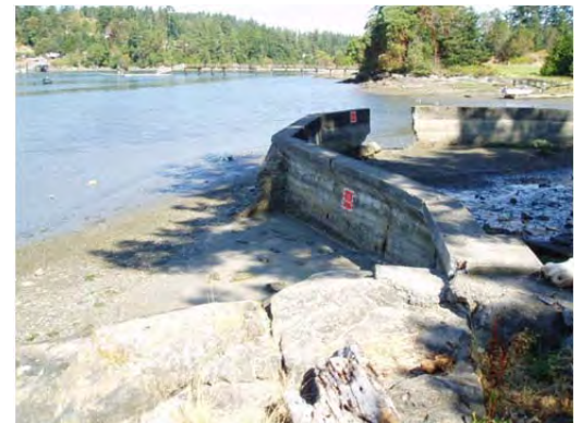
Remains of concrete pool outside pool before removal, looking down-drift in 2006.
