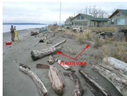
Large wood used to enhance storm berm
