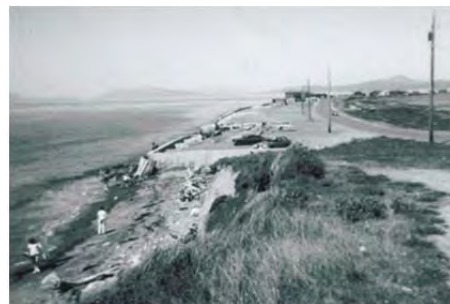
Swan Lake project site in about the early 1970s, looking down-drift. Vertical concrete bulkhead and backfill at up-drift end of study area failed soon after construction.
