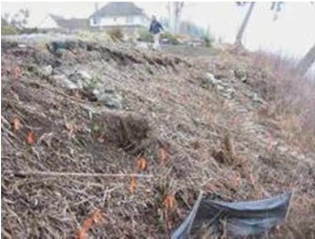
View looking south shortly after cleanup and removal of invasive vegetation and initial planting of native vegetation. Note tension crack at top of slope and slumping of soil and mantle of fill and topsoil.
