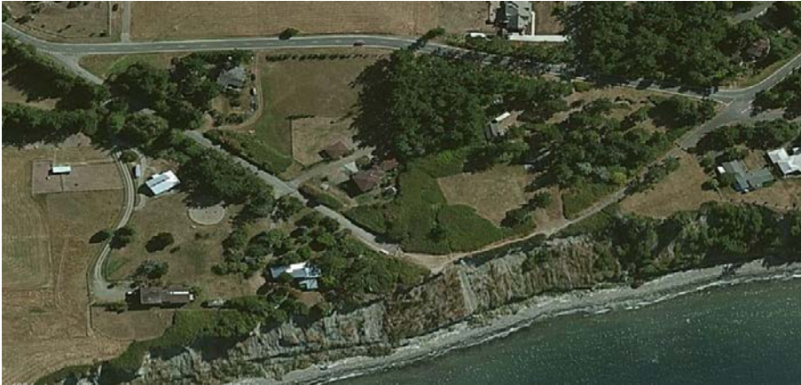
Figure 6-4. Cook Road located northwest of Port Townsend along the Strait of Juan de Fuca. The realigned road is at the top of the photograph and the abandoned road at the bottom where the corner has been cut away by bluff erosion. The narrow, steep beach and high energy waves cause persistent erosion with no backshore to locate a practical bulkhead. The relocation took place in the 1990s (Dept. of Ecology Digital Coastal Atlas).
