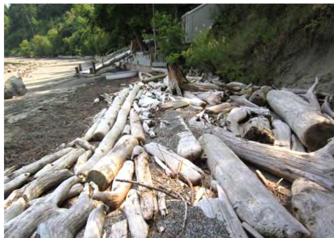
Up-drift beach and vertical soldier pile bulkhead looking down-drift in 2012.
