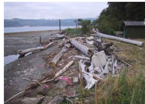
Looking northwest at site in July 2002 prior to the project. Ecology blocks were recently undercut by the stream and wave attack.
