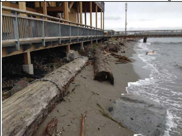
e) Anchored and placed high on the beach for erosion control immediately adjacent to the Northwest Maritime Center in Port Townsend.
