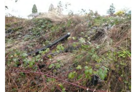
Bluff before treatment. Note drainage pipes and invasive Himalayan blackberries.
