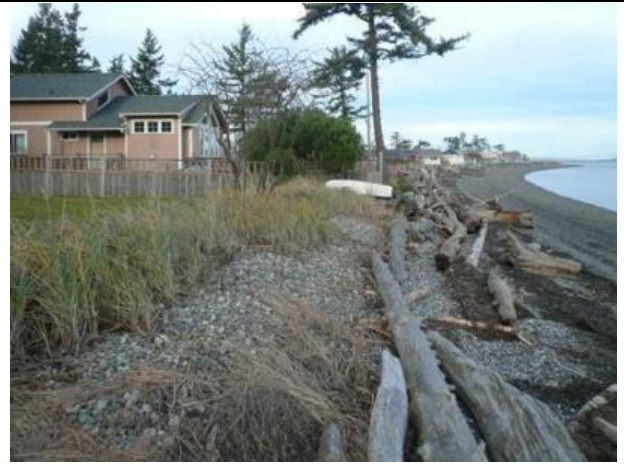
b) East Lummi Island, Whatcom County; MHHW-backshore placement
