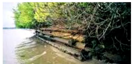
Log bulkhead at the site in 2005 shortly before removal.
