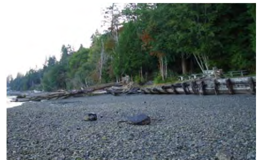
Bulkhead looking north in 2006.
