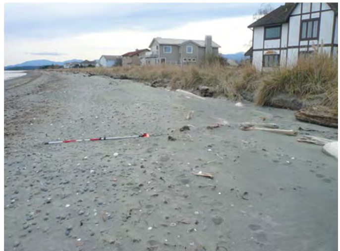
Project site looking southeast. Note dense dune grass growing atop the nourished dune, with some installed berm logs exposed in the foreground.
