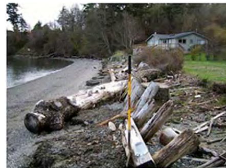
Southward view of the site prior to implementation. Note failed soldier pile wall in the foreground, along with erosion scarp.
