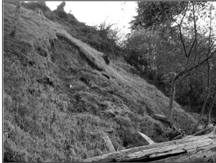
Figure 7.3-5. The slope shown above in unconsolidated sediments was too steep and the roots of the grasses planted too shallow to hold up without some combination of deep-rooted vegetation, contour brush layering, stepped slope contouring, and temporary geotextile or other engineered structure (preferably including vegetation).
