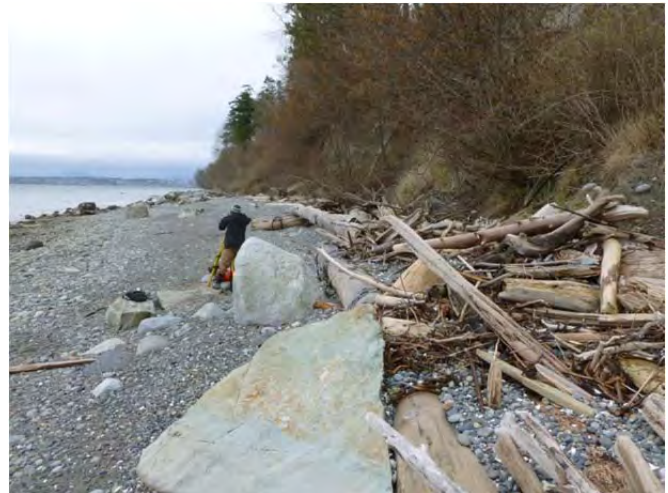
Project site looking down-drift in 2012. Note anchored logs and large accumulation of LWD landward of logs. Boulders were present prior to the project.
