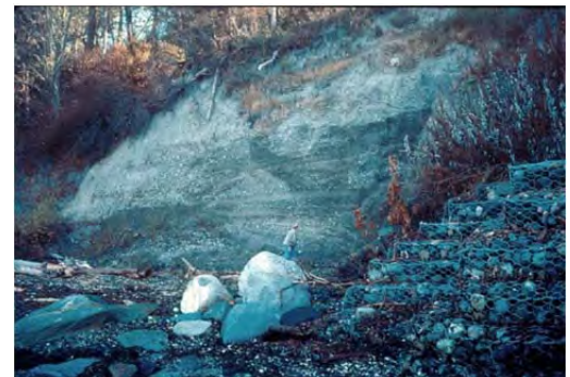
Bluff face devoid of vegetation adjacent to gabion baskets (right). Person for scale above boulders.
