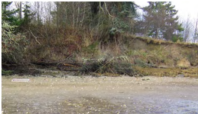
The reach from which the concrete bulkhead (left half of photo) and the pit-run rock bulkhead (right half of photo) were removed. Note the willow growing from the left portion of the bank. Here, the bluff was regraded to a gentler angle and planted with willow stakes. The extent of pickleweed, visible growing in front of the right portion of the bank, appears to have been slightly reduced through burial by eroding sediment since bulkhead removal.
