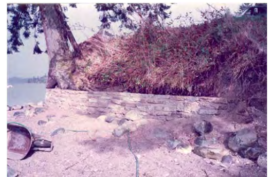
Earlier bulkhead looking northeast in the 1970s.
