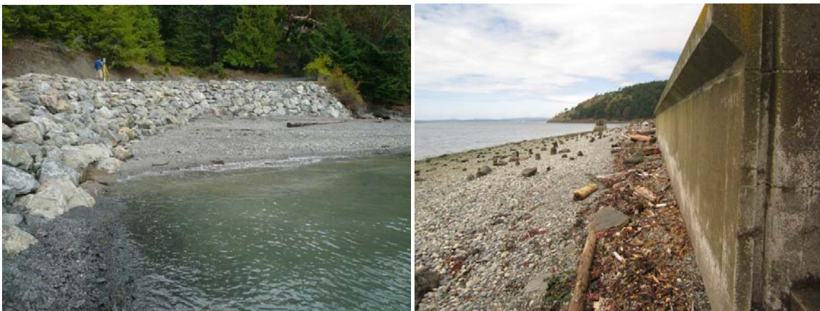
Figure 7.5-1. Photos showing a revetment (left) and vertical bulkhead (right).
