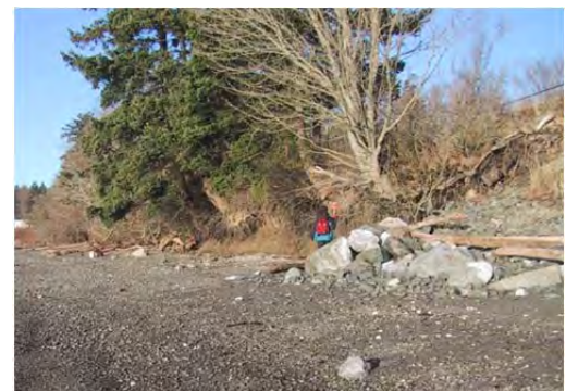
Photo taken in January 2003 of the north end of the project revetment. Degradation—already apparent—began within 2 years of installation.
