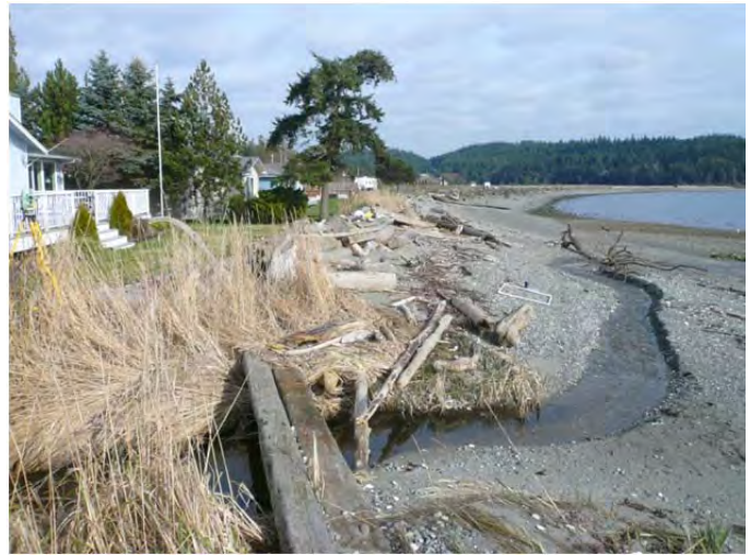
Looking down-drift in 2012. South log is visible behind dunegrass.
