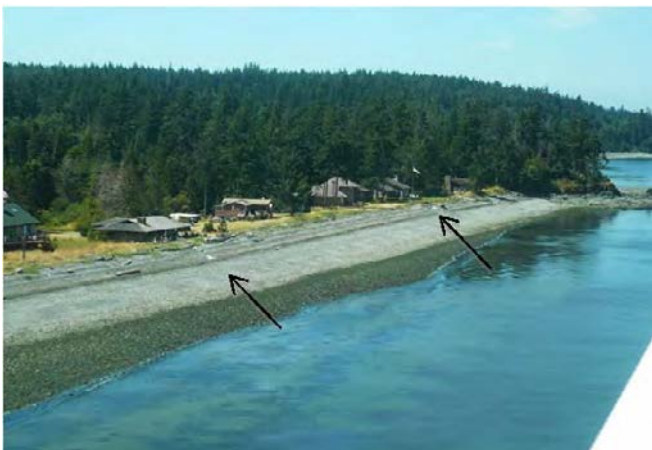
Project area in 2008 with drift sills (at arrows) barely visible on uppermost beach.
