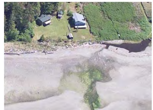
Looking northeast to site in May 2001 prior to construction (Washington State DOE photo).
