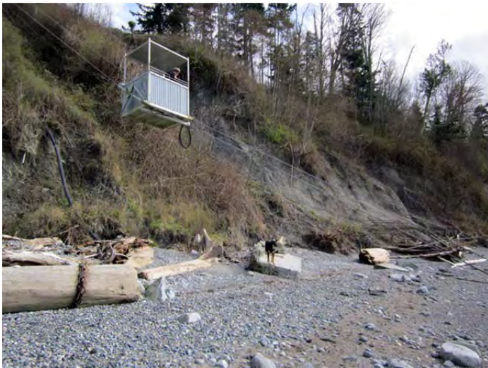
Gabion bulkhead removal area in 2012. Note extensive recent landslides both on site and farther south (up-drift), as well as remaining concrete debris.
