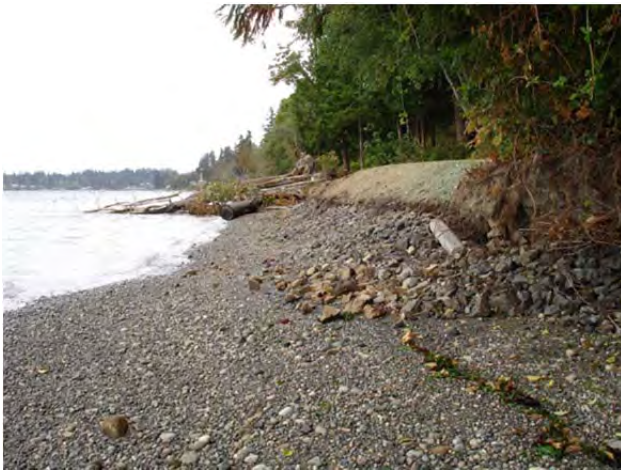
Photo looking north taken shortly after the bulkhead was removed looking northeast. Quarry spall was left on site. The steep bank was regraded and seeded with grass.
