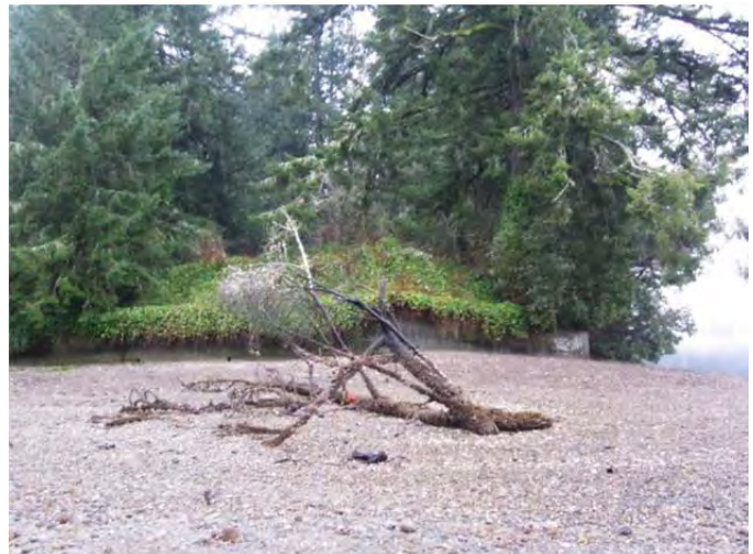
Bulkhead looking southeast from the point of Snyder Point in 2012.
