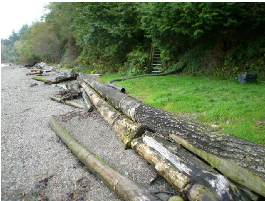
Figure 7.2-5. Example of inappropriate large wood project on south Whidbey Island which was constructed with fixed, stacked logs placed lower and more vertically than designed or permitted, here retaining fill gravel and creating usually dry land where beach existed prior.
