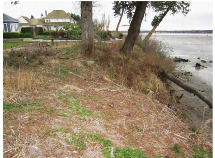
Looking south over treatment site where nonnative plants were removed and upper bank was replanted with native plants in 2012.
