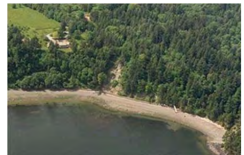
Oblique 1994 aerial view with an older bulkhead present. Large landslide visible in east-central bulkhead area, with smaller failure to right.
