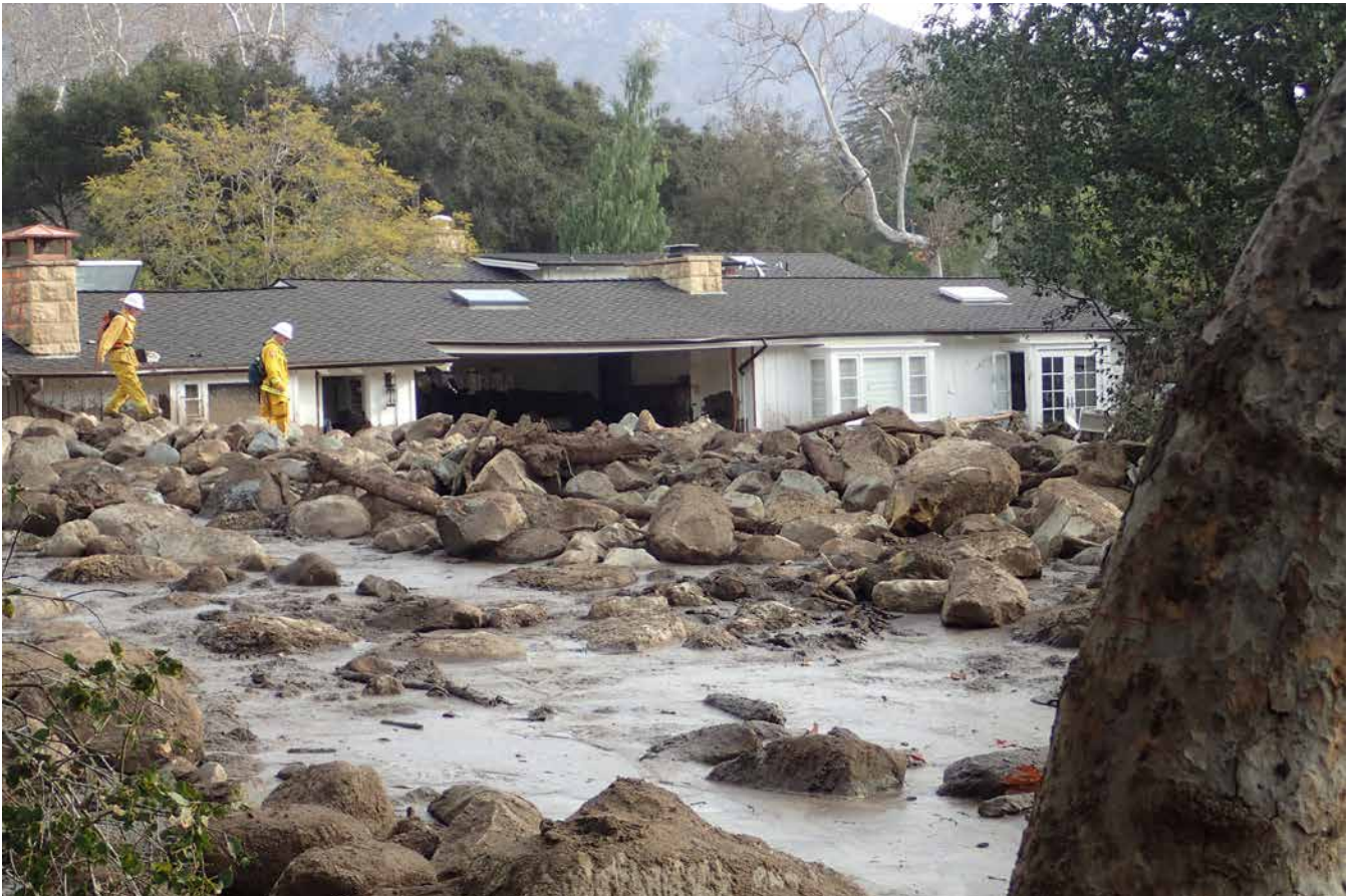
Figure 3.8. Heavy rains one month after a series of major wildfires in 2018 resulted in a mudslide in Montecito, California that caused 23 deaths.
