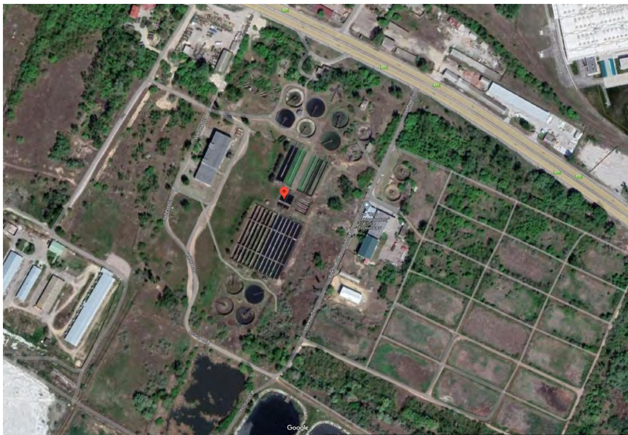
Figure 49. Oleshki wastewater treatment plant (Source: Map data @2023 Google)
