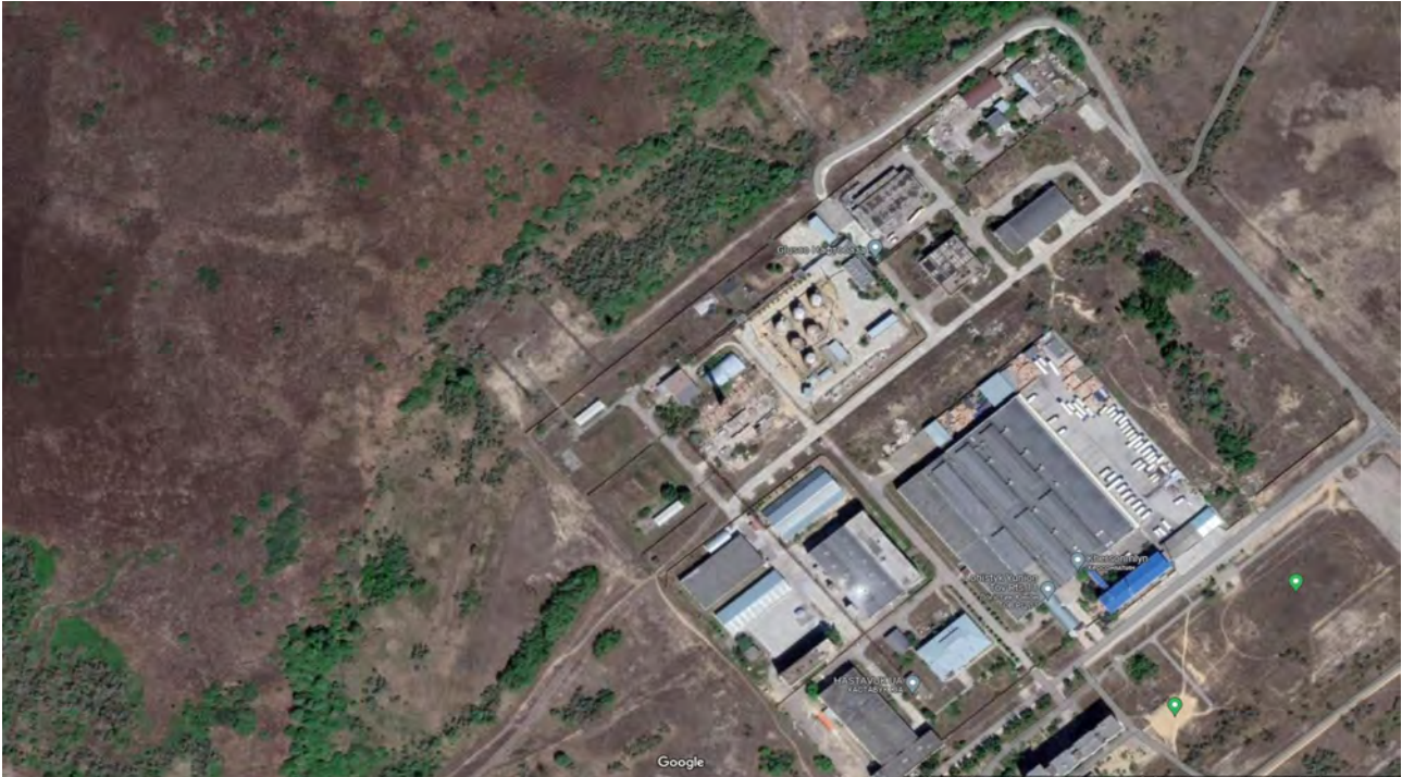
Figure 45. Glusco fuel storage area (Source: Map data @2023 Google)
