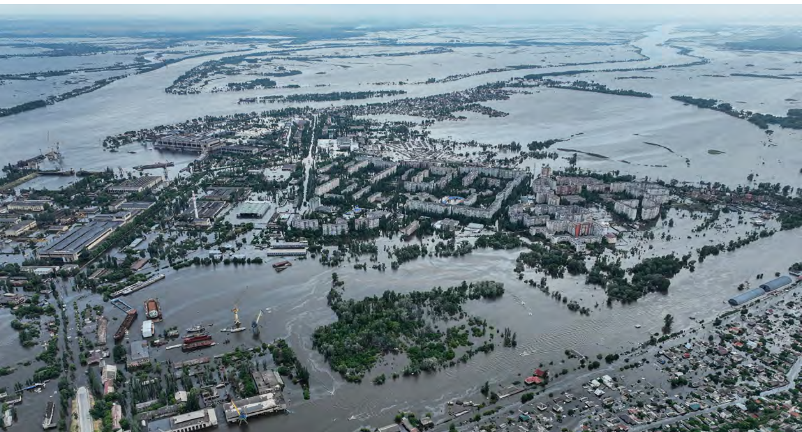
Figure 31. The photo taken on 10 June 2023, shows flooded area west of Kherson on the northern side of the river. Heavy industry and residential areas are located close together (© KEYSTONE/ AP Photo)
