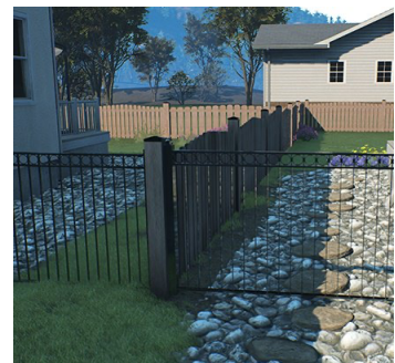
Combustible fences when ignited can provide a pathway for fire to reach your home.
