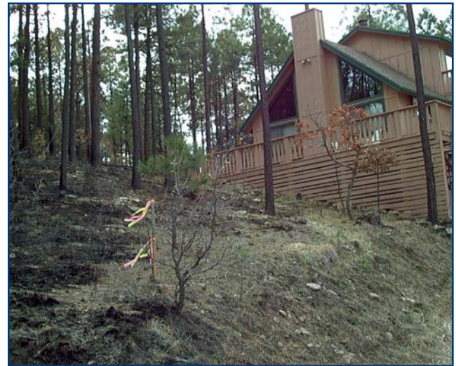
The pre-fire activities implemented by this homeowner include a maintained landscape, use of Firewise plant materials, reduced vegetation around the perimeter of the property and fire-resistant roofing material.
