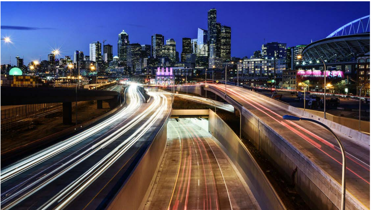
SR 99 tunnel (WSDOT)
