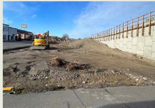
Lewis Street Bridge Overpass, Pasco, WA.
