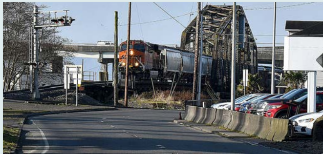
US 12 Highway-Rail Grade Separation in East Aberdeen
