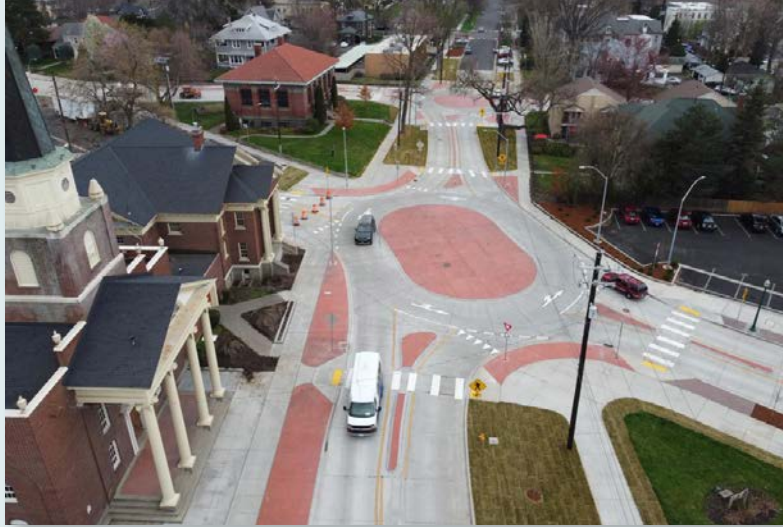
Roundabouts at the intersections of Alder/Park, Alder/Palouse, and Poplar/Palouse in Walla Walla
