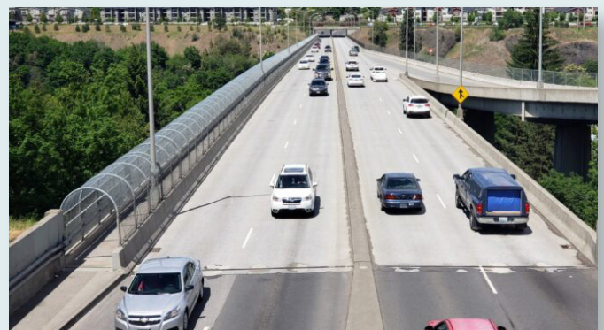
Maple Street Bridge deck replacement in Spokane
