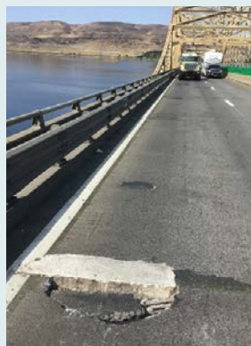
I-90 Vantage Bridge Deck Replacement
