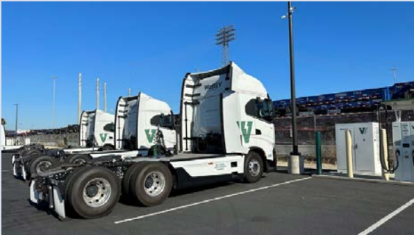
WattEV public truck charging depot in California
