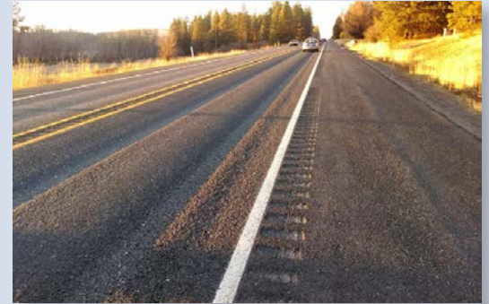
Studded Tire Wear, State Route 904 North of Cheney
