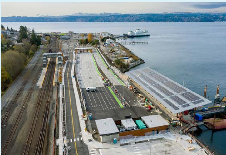
Mukilteo Ferry Terminal
