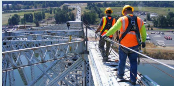
Lewis and Clark Bridge, State Route 433 spanning the Columbia River
