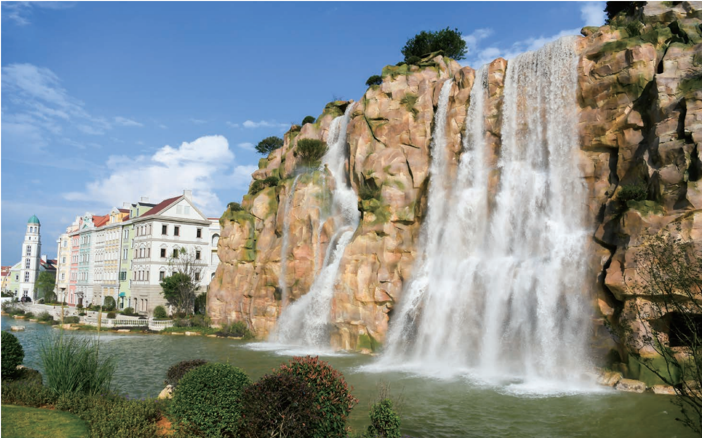
Huawei Cloud's green data center in Gui'an: Naturally cooled through direct ventilation and by waterfalls and lakes, with an industry-leading PUE of 1.12
