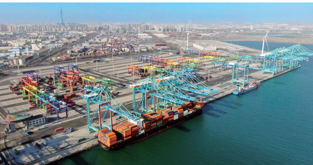
The Port of Tianjin has chosen Huawei to support its digital transformation. It aims to constantly improve its levels of automation and intelligence and become a smart, green, and safe port.
