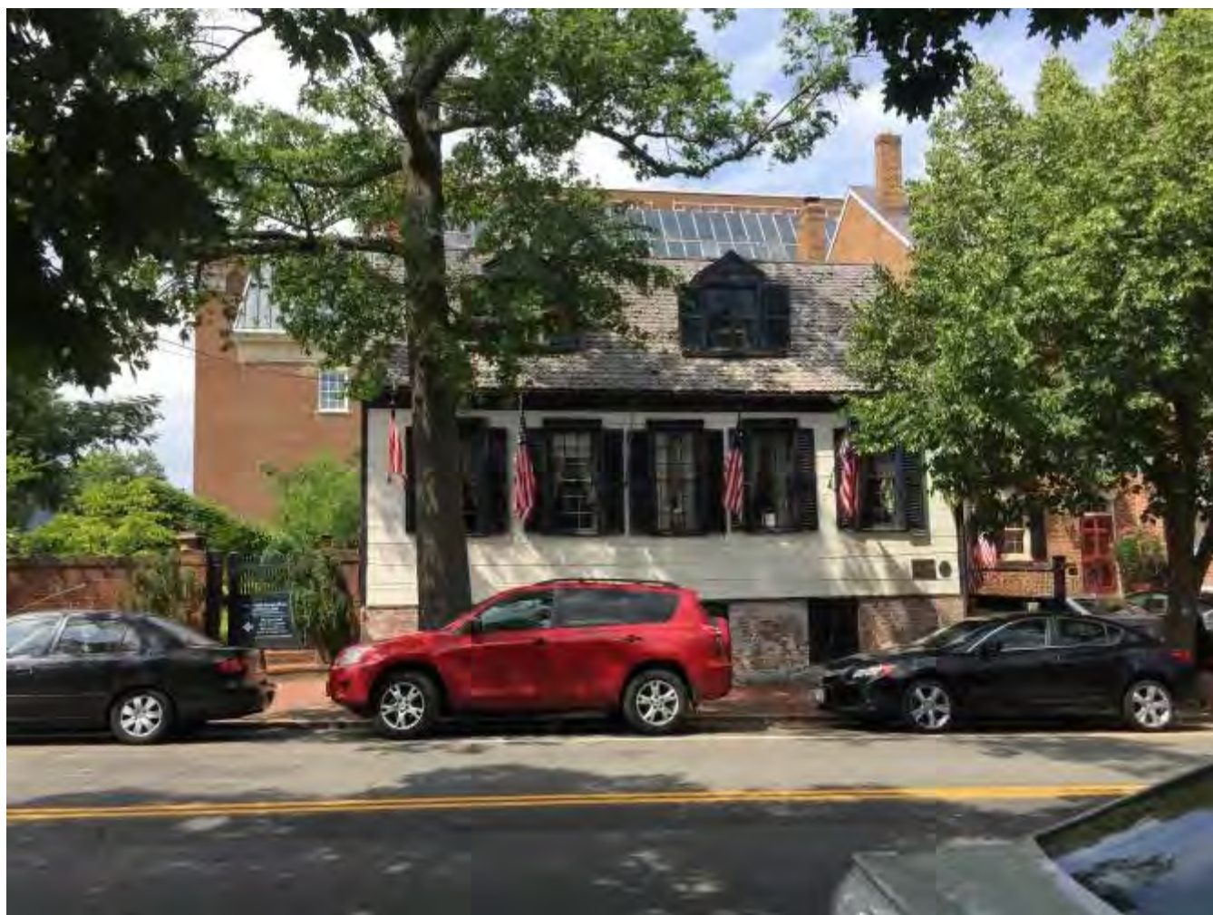
2 of 7. Murray-Dick-Fawcett House, south elevation.
