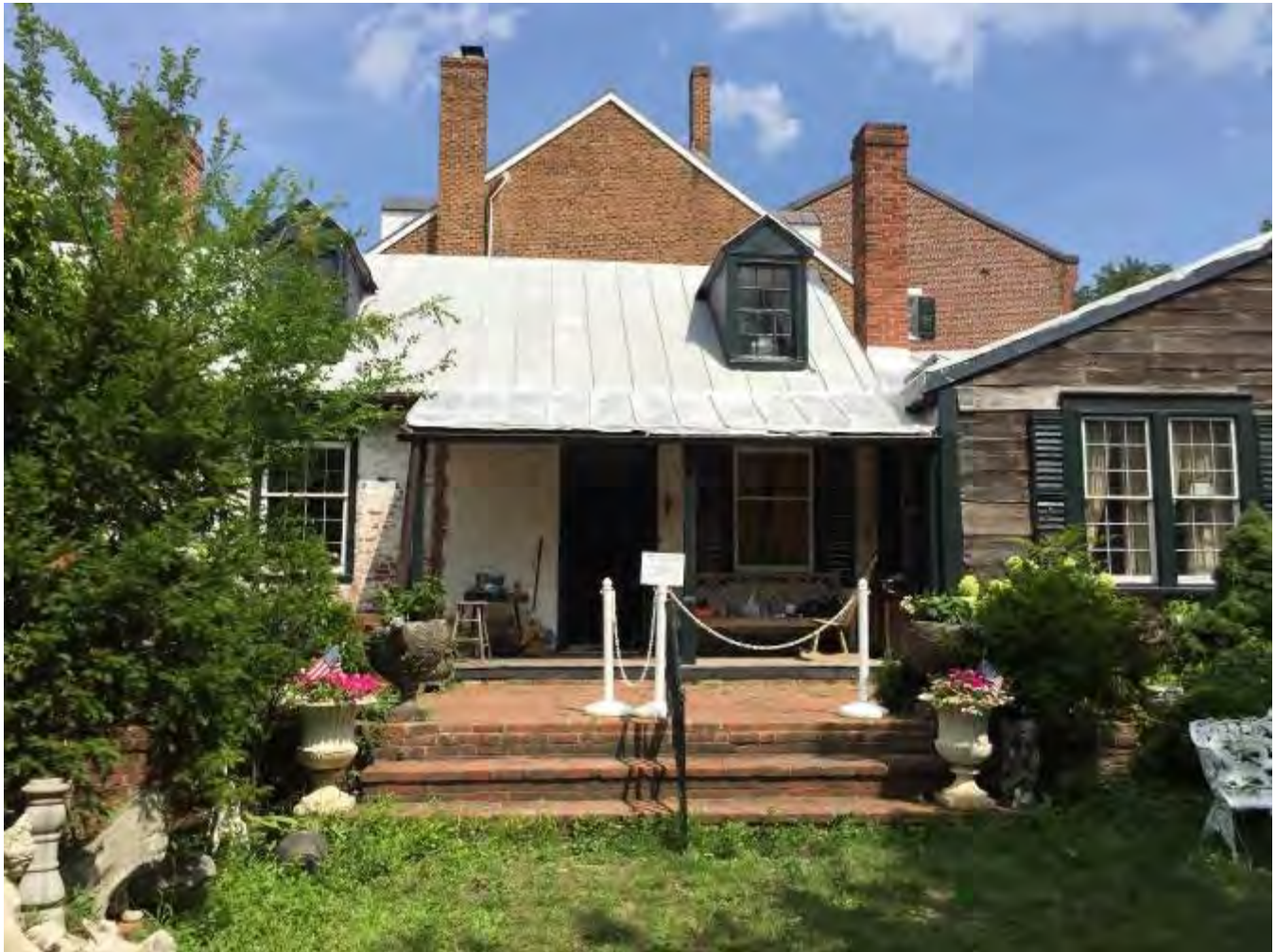
5 of 7. Murray-Dick-Fawcett House, west elevation of north additions.
