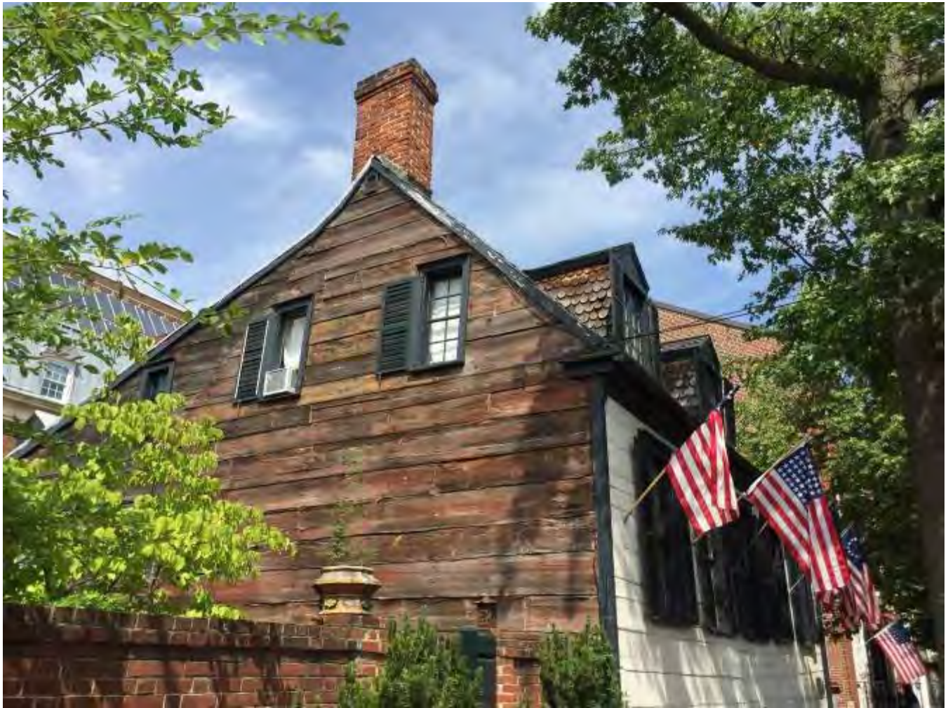
3 of 7. Murray-Dick-Fawcett House, west elevation.
