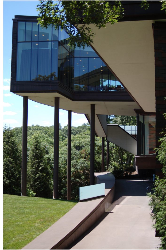
COLUMN AT CANTILEVERED CORNER
