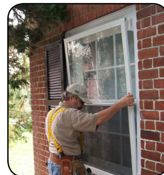
Installation of an exterior storm window.
