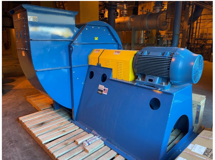
Figure 2: New Over Fire Air Fan – Boiler No. 3 LN™ Technology Installation
