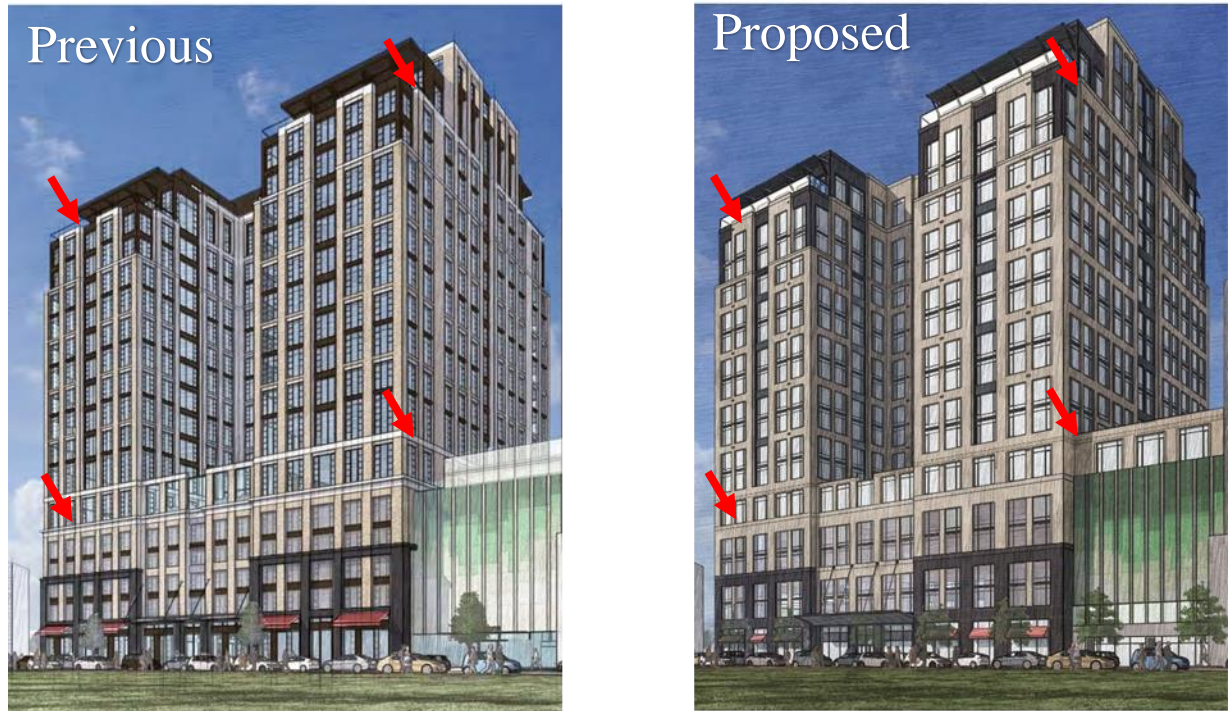
Figure 16: Staff find the previously approved the cast-stone trim to be desirable feature, which was effective in enhancing the perception of the tower as a three-dimensional building.
