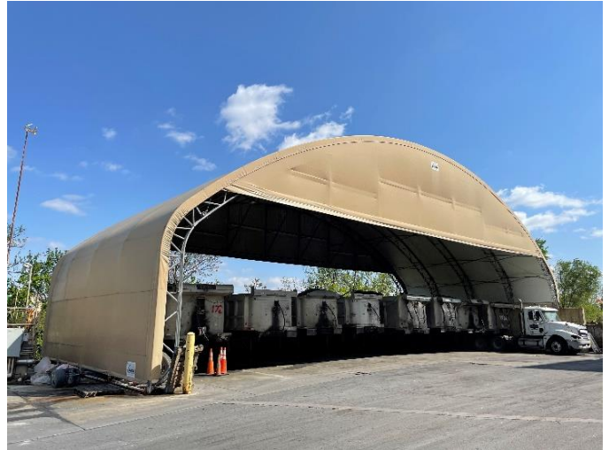
Figure 14: Ash Trailer Canopy
