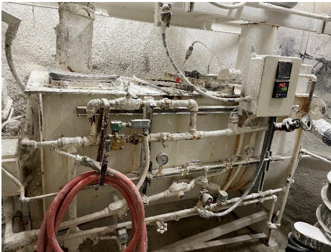
Figure 33: Pebble Lime Slaker
