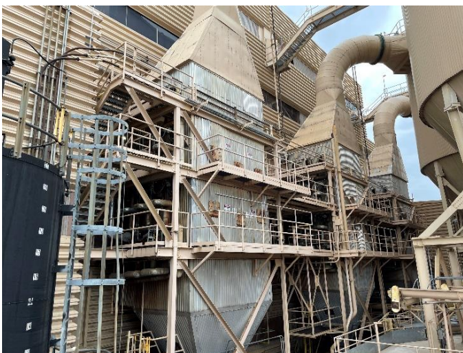
Figure 29: Boiler Economizer
