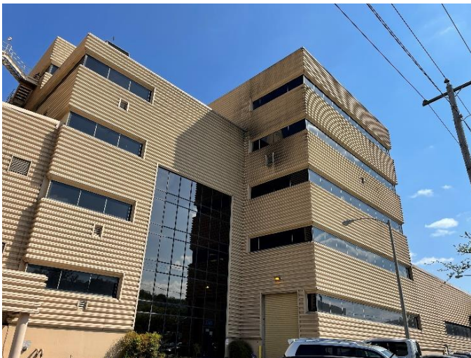
Figure 11: Front side of Facility (view from Eisenhower Ave.)
