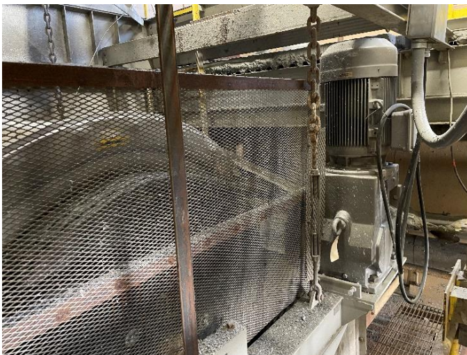
Figure 5: New VFD (variable frequency drive) for the magnet
