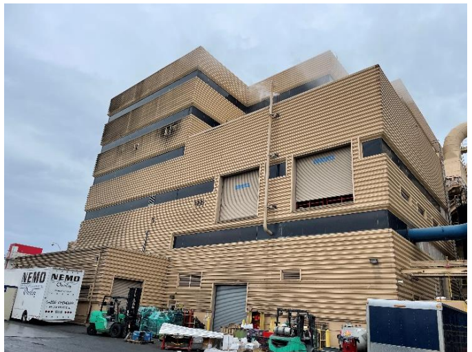
Figure 12: Back side of Facility
