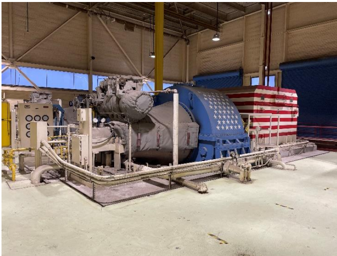
Figure 27: Turbine-Generator
