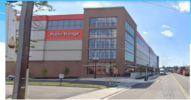
Recent industrial building constructed on Pickett Street
