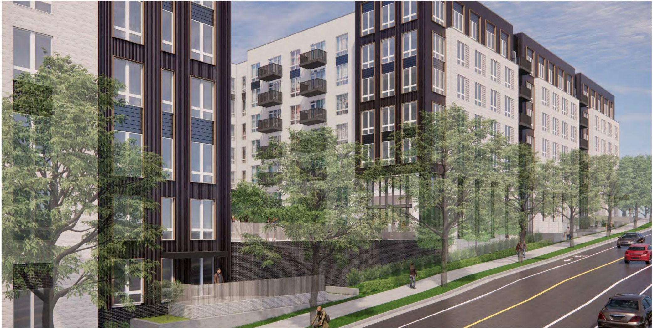
view of amenity and courtyard on stevenson ave.
