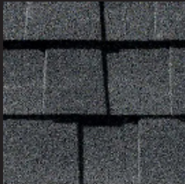
^ ARCHITECTURAL GRADE ASPHALT 20TH - 21ST CENTURY
