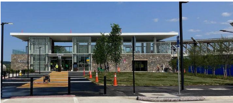
Image: PY Metro Station North Pavilion
