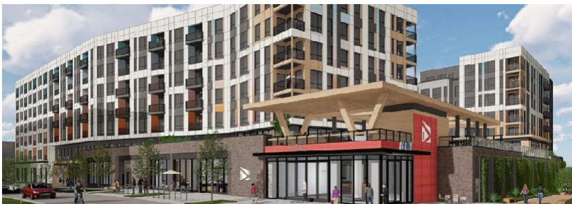
View of the Southwest corner of the Block I building.
