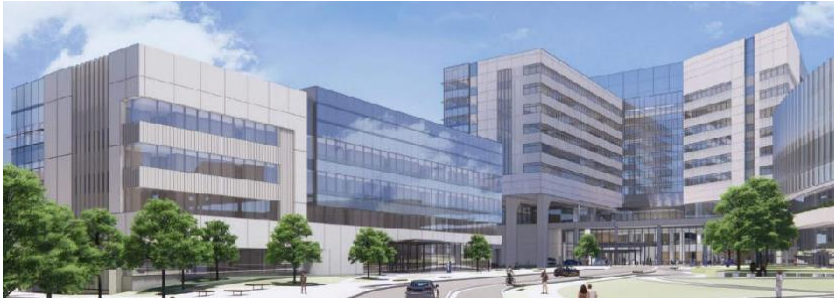
Figure 1 Inova Hospital Campus viewed from West End Blvd. looking West.
