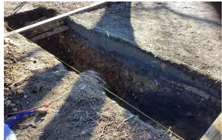
Photo of existing utility trench by Gray and Pape
