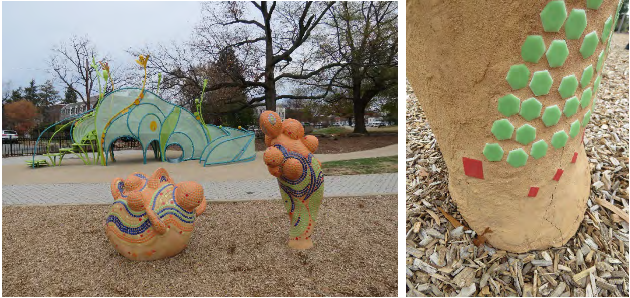
(Left) The public artwork consists of three main components, including a large climb-on structure, two mosaic sculptures, and an entrance gate. (Right) Cracking at the base of the mosaic sculpture.
