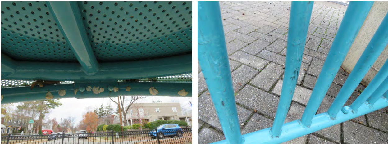
(Left) Numerous stickers and remnants of stickers are present on the underside of the large climb-on structure. (Right) Scuff marks and abrasions are seen at the base of the gate.
