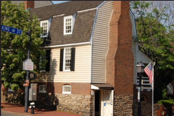
The stone foundation of the 18th-century Ramsay House shows the original height before King Street was regraded.
