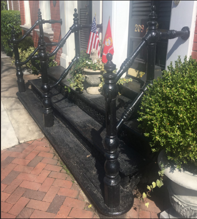
Example of historically appropriate cast iron steps and handrail on an Italianate style residence.
